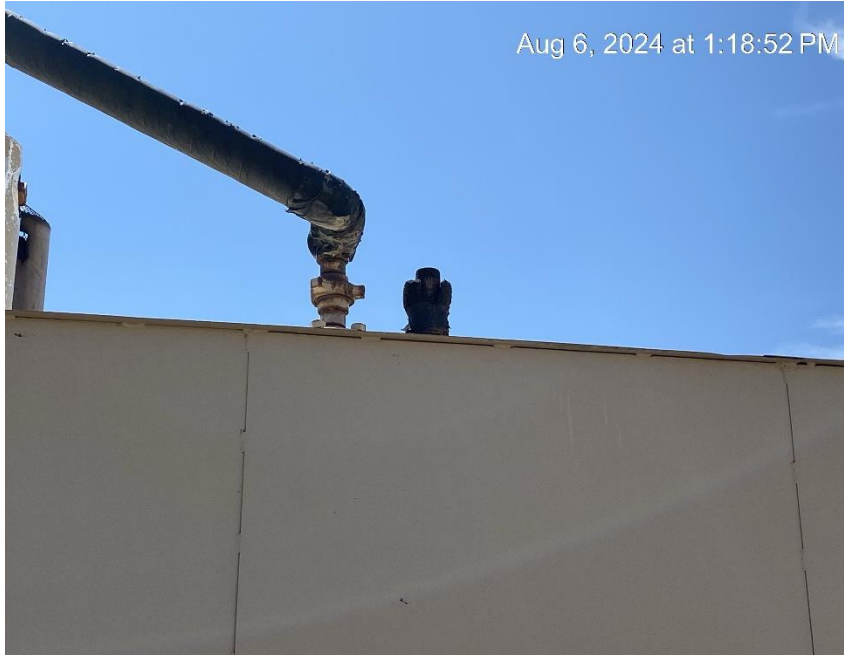
Relief riser missing protective cap
