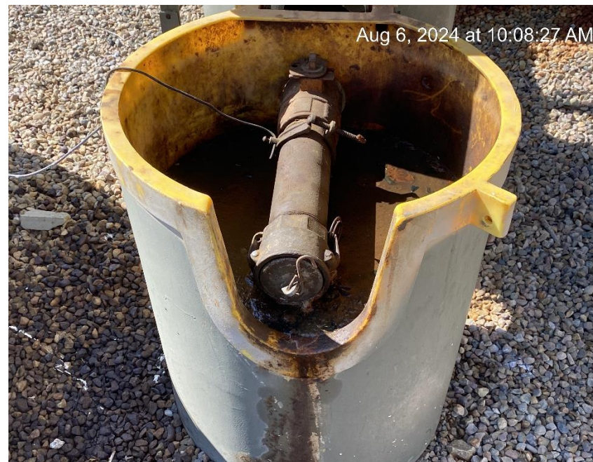
Cap drip. Valve open inside pot.
