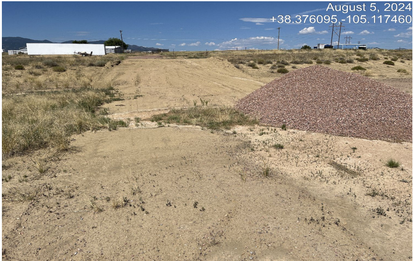
Photo 6. Facing west toward the cut slope which is not stabilized. There is new disturbance in this area.
