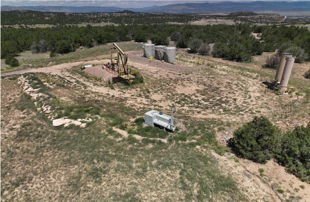
Photo 4. Facing northwest. This well has been inactive for a long period of time. Equipment is unused and needs to be removed. There are weeds growing around the equipment which is a fire hazard.
