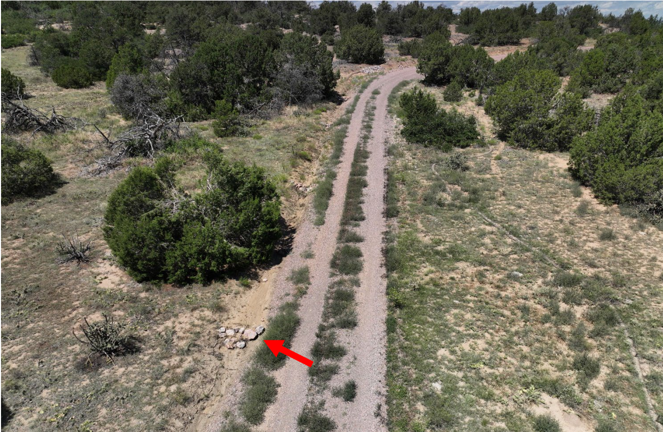
Photo 1. Drone aerial photo facing northwest along the access road. There are some check dams where stormwater is going around the check dam. BMP maintenance is needed. Previous corrective action was not completed.
