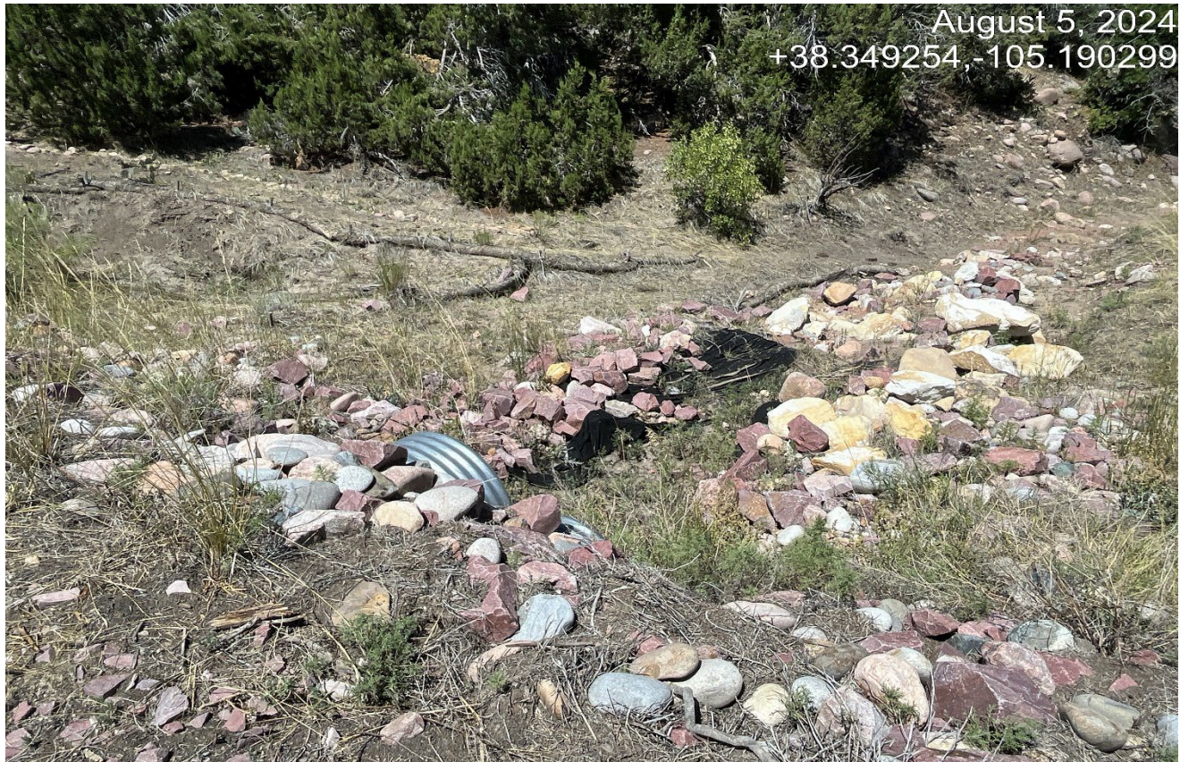
Photo 2. View of culvert outlet shows displaced rock. Outlet protection will need to be reinstalled. Previous corrective action was not completed.
