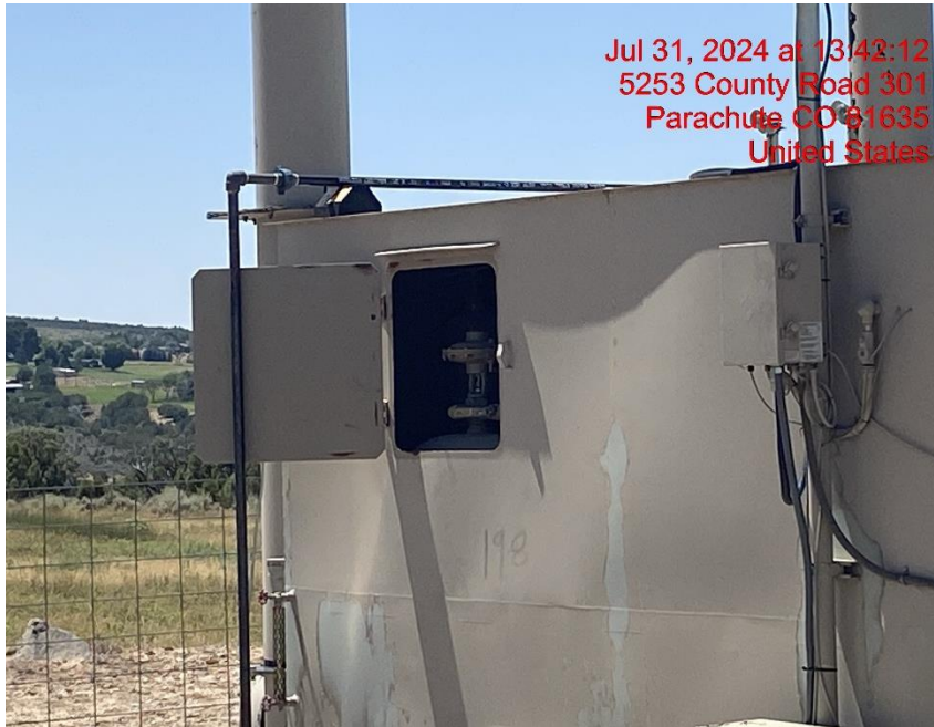
Unsecured Separator – Photo #02576
