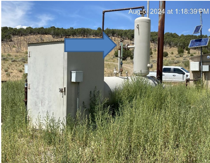
Weeds. Relief risers missing caps
