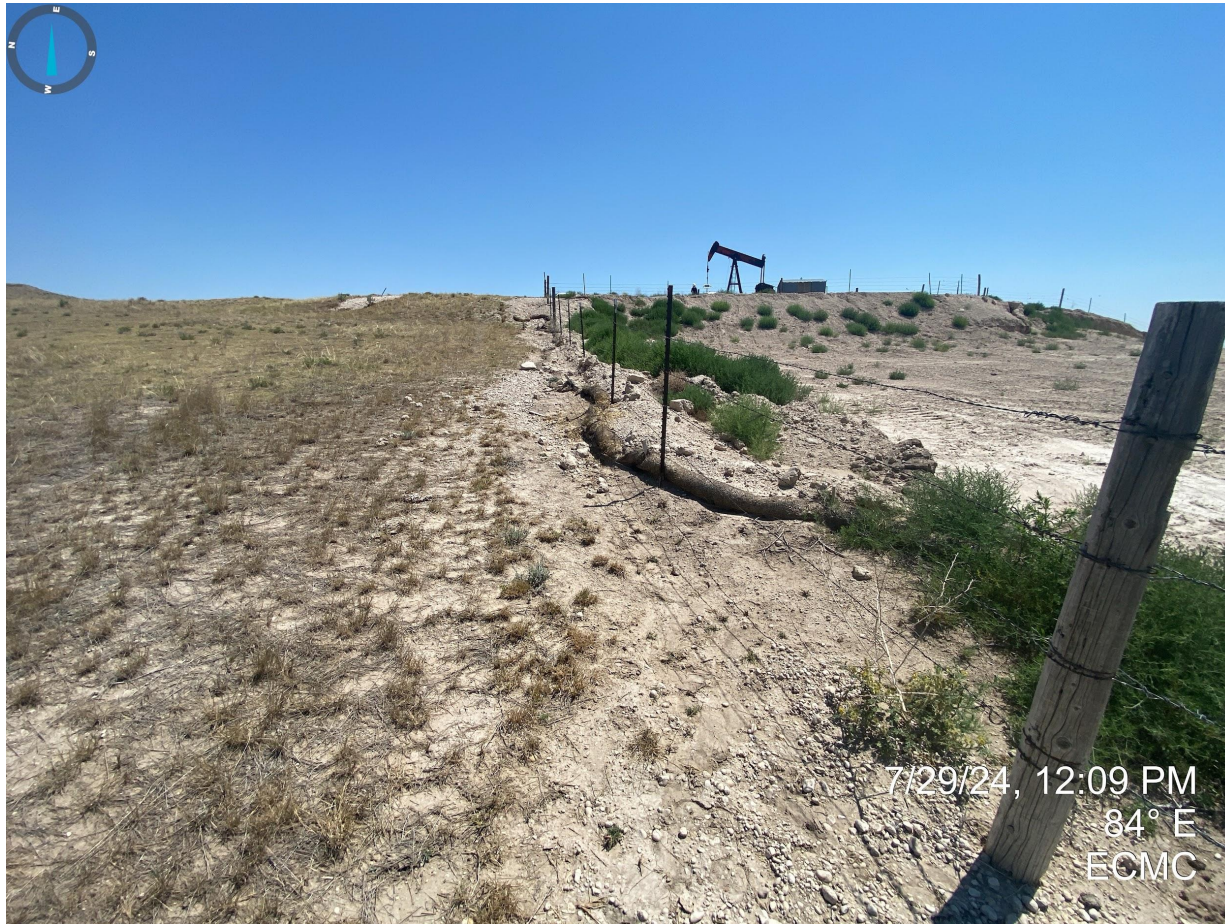
Photo 21. Taken from the north side of the pit. It does not appear that any erosion degradation has been properly stabilized or repaired, and stormwater control measures remain inadequate as the straw wattles are degraded and not properly functioning
