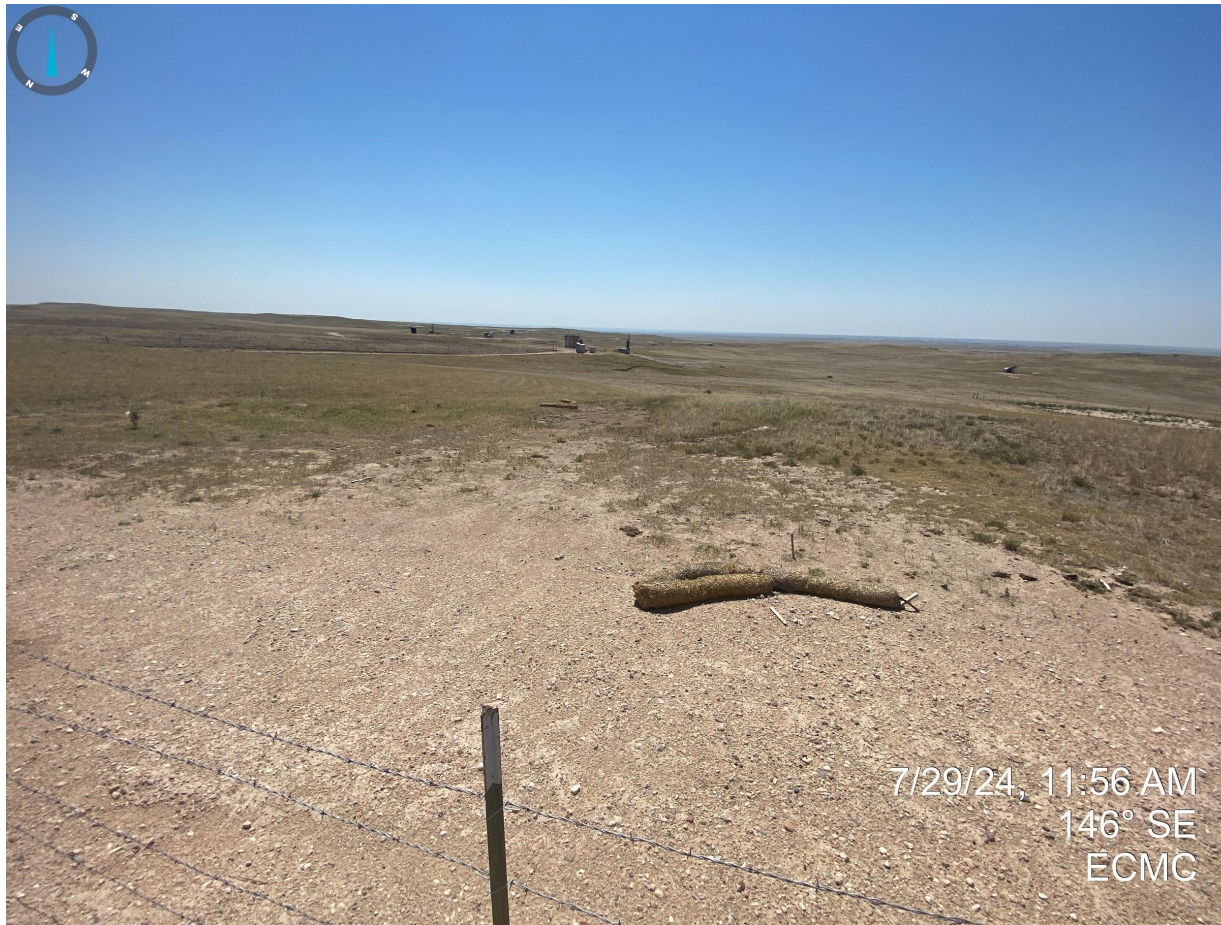
Photo 5. Facing southeast at the former heater treater (removed at the time of this inspection). Stormwater control measures (straw wattles) do not appear to be installed per good engineering practices (trenched and backfilled) and require maintenance and or replacement.
