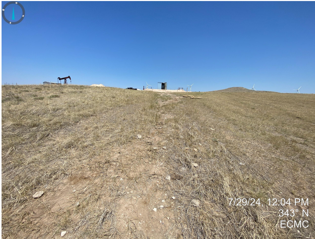
Photo 7. South of the former location of the vertical heater treater. Photo illustrates unstabilized soils and lack of proper stormwater controls measures that would prevent erosion degradation. Sediment deposition observed.
