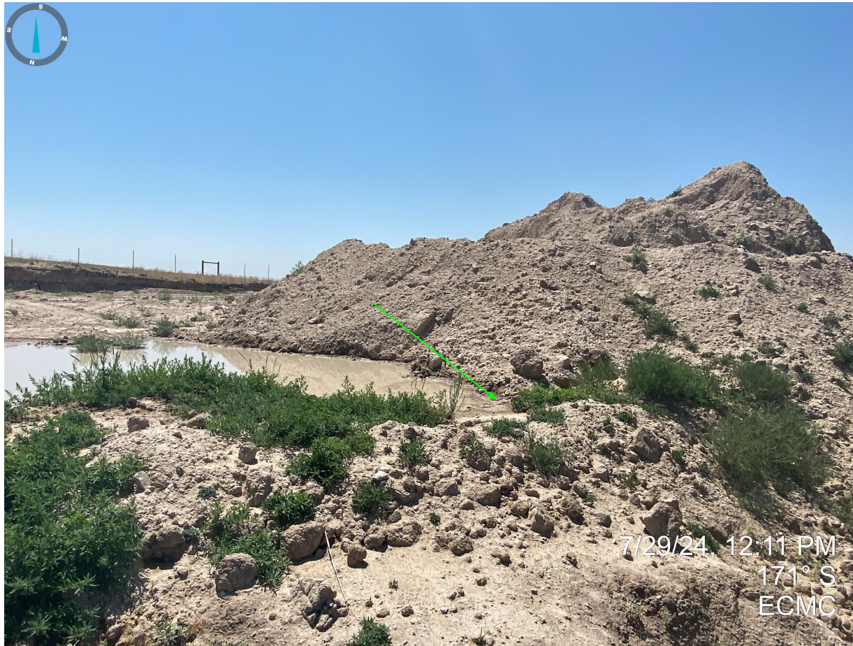
Photo 20. No stormwater control measures/BMPs were observed around the perimeter of the excavated area or stockpiles that would prevent off location stormwater discharge from entering nearby drainage. Stormwater is close to spilling over the excavated area; there is approximately 3 inches of free board (indicated by green arrow).
