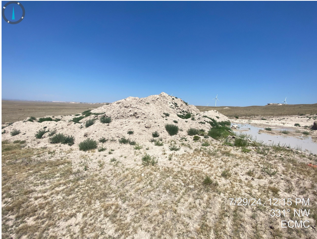
Photo 17. Western stockpiled material is not properly stabilized with evidence of unconsolidated materials. No perimeter stormwater control measures observed.
