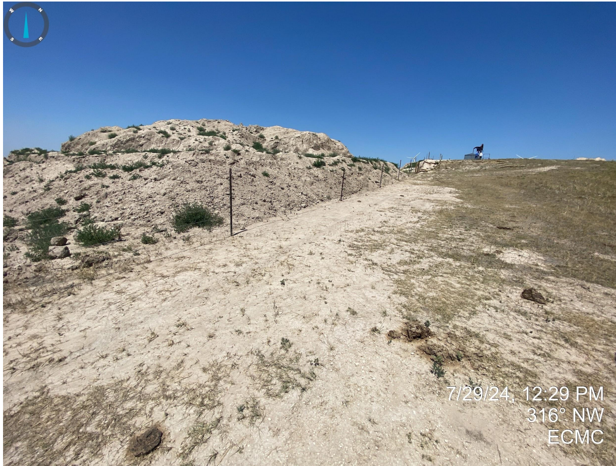
Photo 14. East side of stockpiled pit soils. Photo illustrates that both the stockpile and berms have been left unconsolidated. Unconsolidated materials can become a potential pollution source as it is not properly stabilized. Berms also appear to be built out of impacted material from the salt kill/pit excavation.
