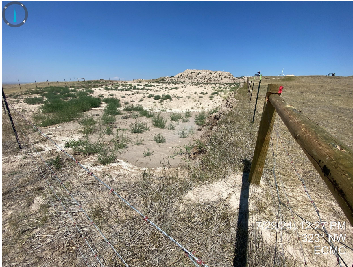
Photo 15. Southern excavated areas do not have any evidence of perimeter stormwater control measures and undesirable vegetation (russian thistle and kochia) was observed growing throughout.
