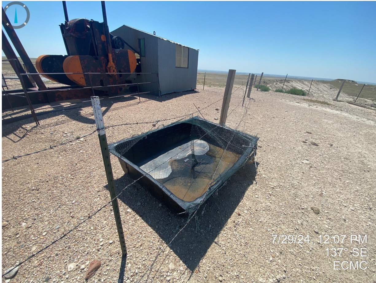
Photo 10. Secondary containment at wellhead does not appear to be in use.
