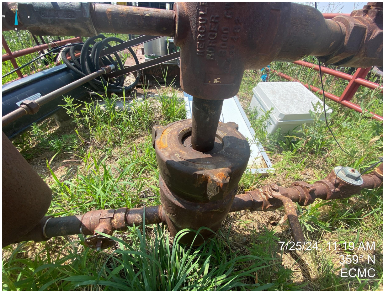
Photo 1. Wellhead casing appears to have been repaired; no visible or auditory indications of venting equipment observed at the time of this inspection.
