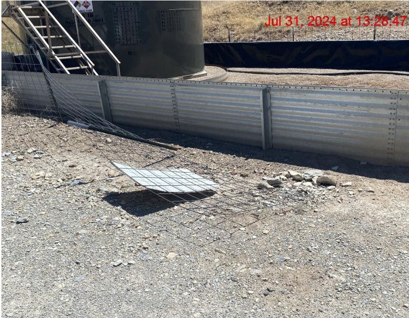
Damaged Battery Fencing – Photo #02565
