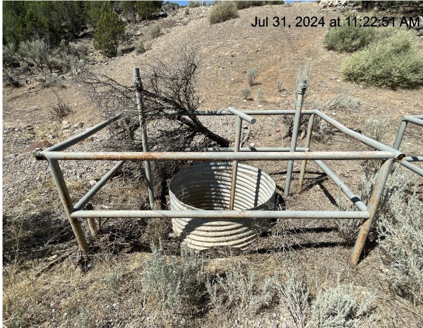
Photo # 4133 Cellar lacks cover/open to entry by wildlife /wildlife hazard (on lease road approximately 75 yards from entrance to location)
