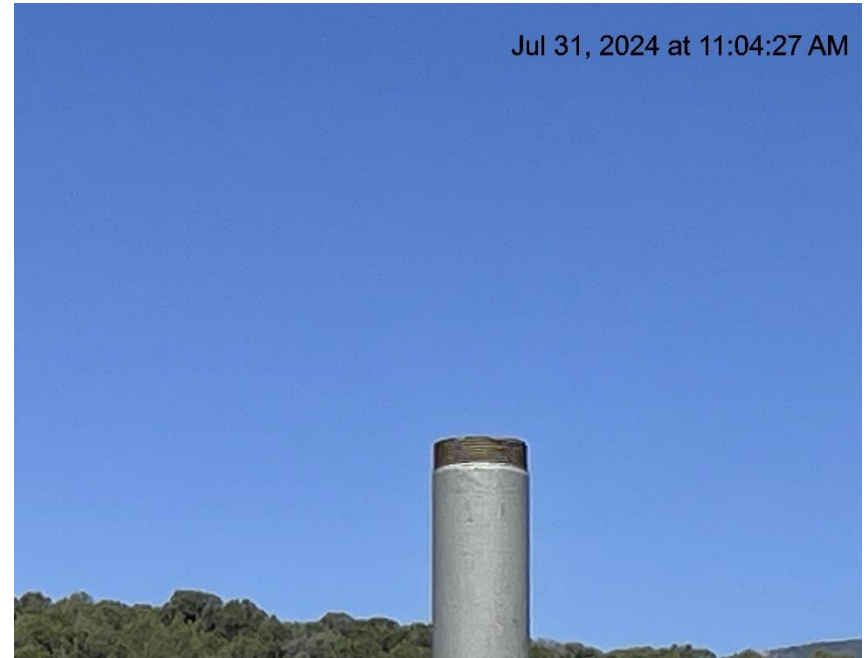
Photo # 4130 Open ended piping on methanol tank/wildlife hazard
