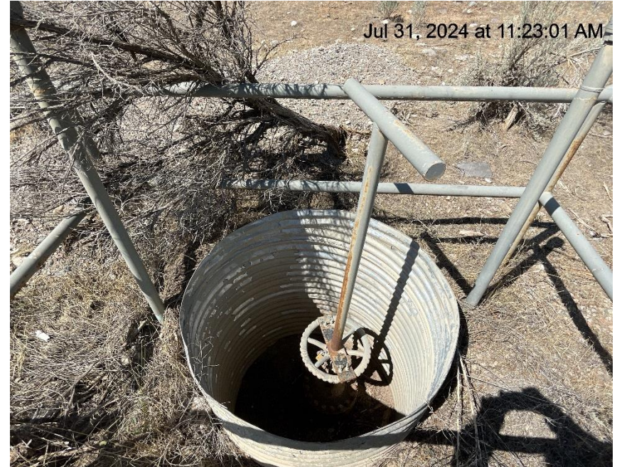
Photo # 4134 Cellar lacks cover/open to entry by wildlife /wildlife hazard (on lease road approximately 75 yards from entrance to location)
