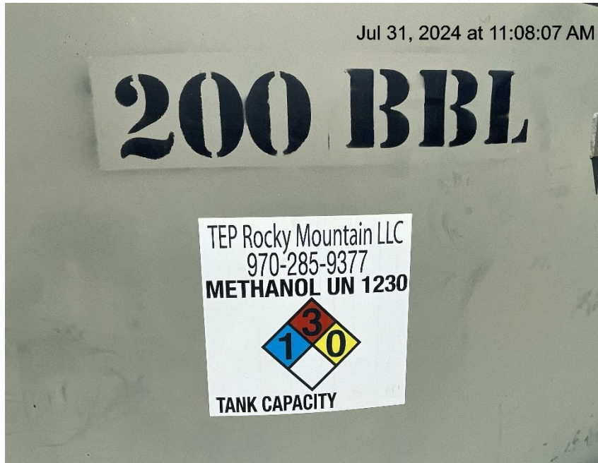
Photo # 4131 Incorrect capacity on methanol tank
