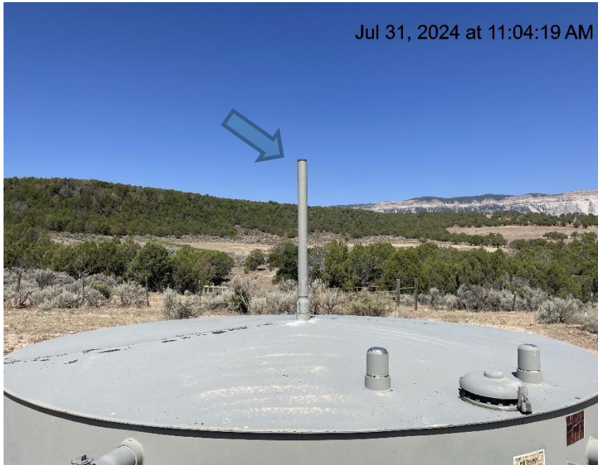
Photo # 4129 Open ended piping on methanol tank/wildlife hazard
