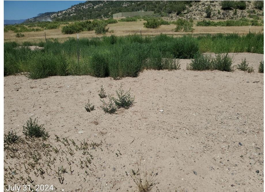
**Photo 2:** Photos 2-3 taken from the southwest end of the Location. Photos provide an overview from southwest, west, north to northeast. production and surface equipment have been removed from the Location; no other reclamation work including, but not limited, removal of gravel, compaction alleviation, recontouring/regrading, replacement of topsoil and revegetation activities have been performed.
