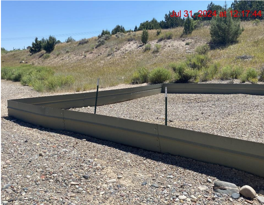
No Berm Liner Installed – Photo #02500
