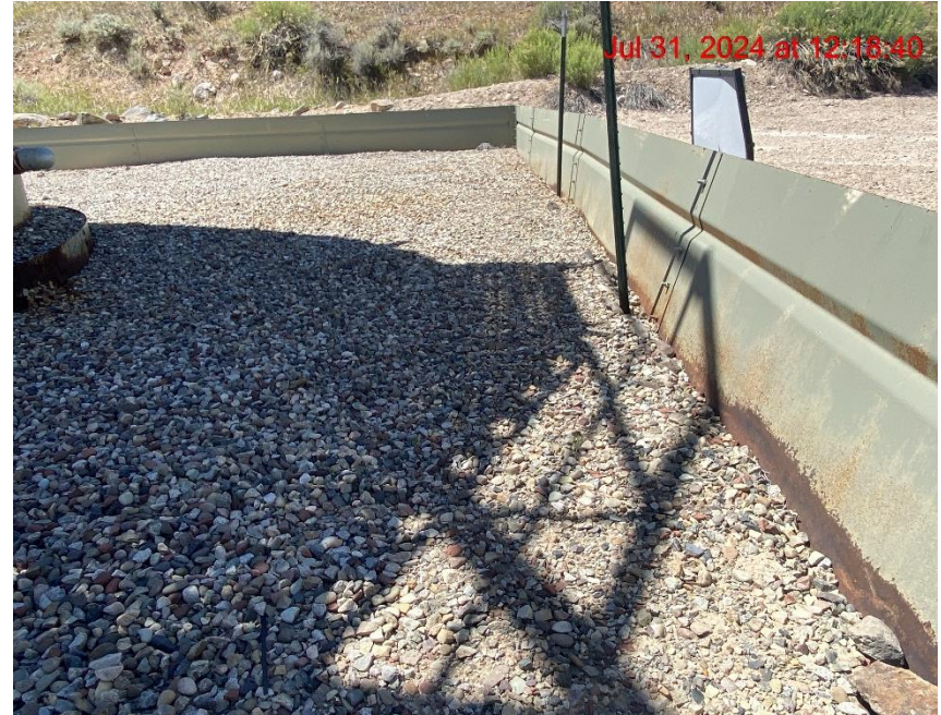
No Berm Liner Installed – Photo #02501
