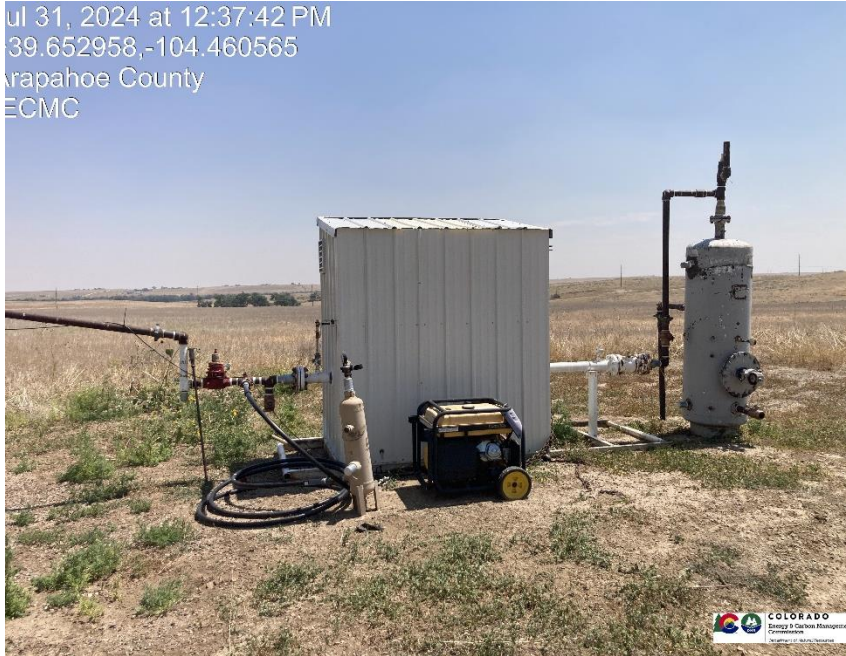
Pic 3 GMR, gas generator, separator.
