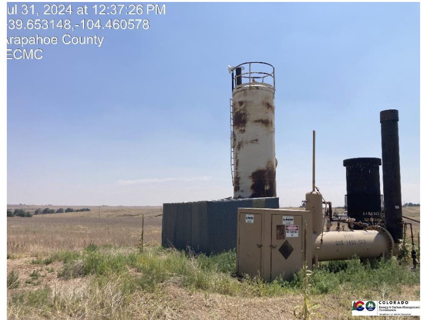
Pic 2 Separators, ECD, weeds unmanaged
