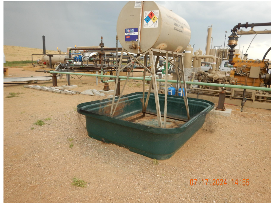
Photo 12. Photo taken along the southern production area, facing South. Photo illustrates wildlife protection devices (netting) are present for secondary containment BMPs.
