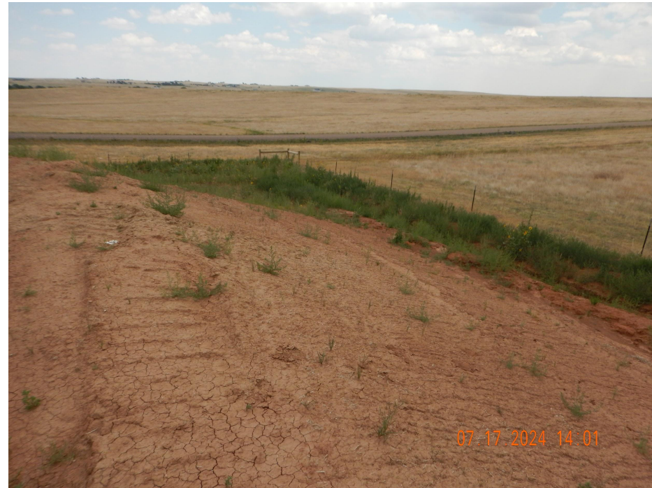
Photo 2. Photo taken along the southeastern working pad surface, facing East. Photo illustrates the reclamation construction areas appears to have been repaired from stormwater erosion. Note- tumbleweed is establishing along the perimeter of the location.
