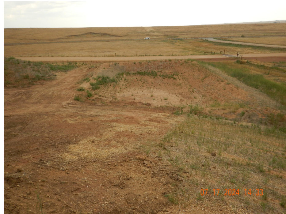
Photo 10. Photo taken along the northeastern working pad surface, facing North. Photo illustrates a retention pond and areas appears to have been repaired from stormwater erosion.
