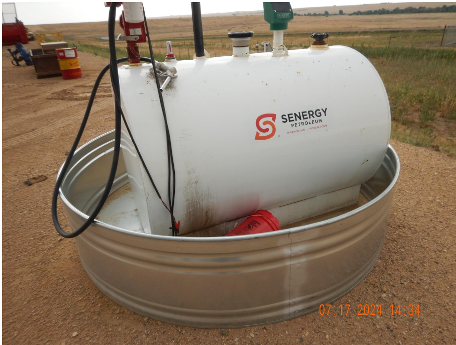
Photo 11. Photo taken along the eastern working pad surface, facing Northeast. Photo illustrates wildlife protection devices (netting) are missing for secondary containment BMPs.
