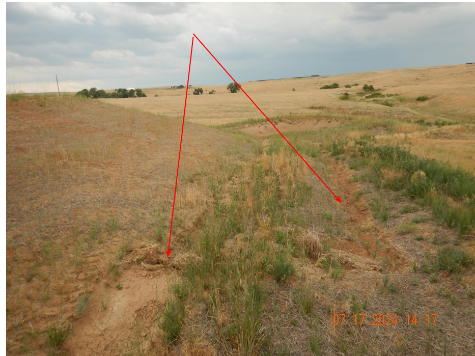
Photo 6. Photo taken along the western perimeter of location, facing West. Photo illustrates straw mulch blockage in the ditch BMP directed to the retention pond; this resulted in stormwater erosion bypassing the retention pond but mostly staying within the outer perimeter berm BMP.
