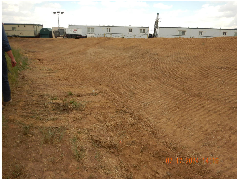
Photo 7. Photo taken along the western perimeter of location, facing East. Photo illustrates slope tracking has not been implemented properly.
