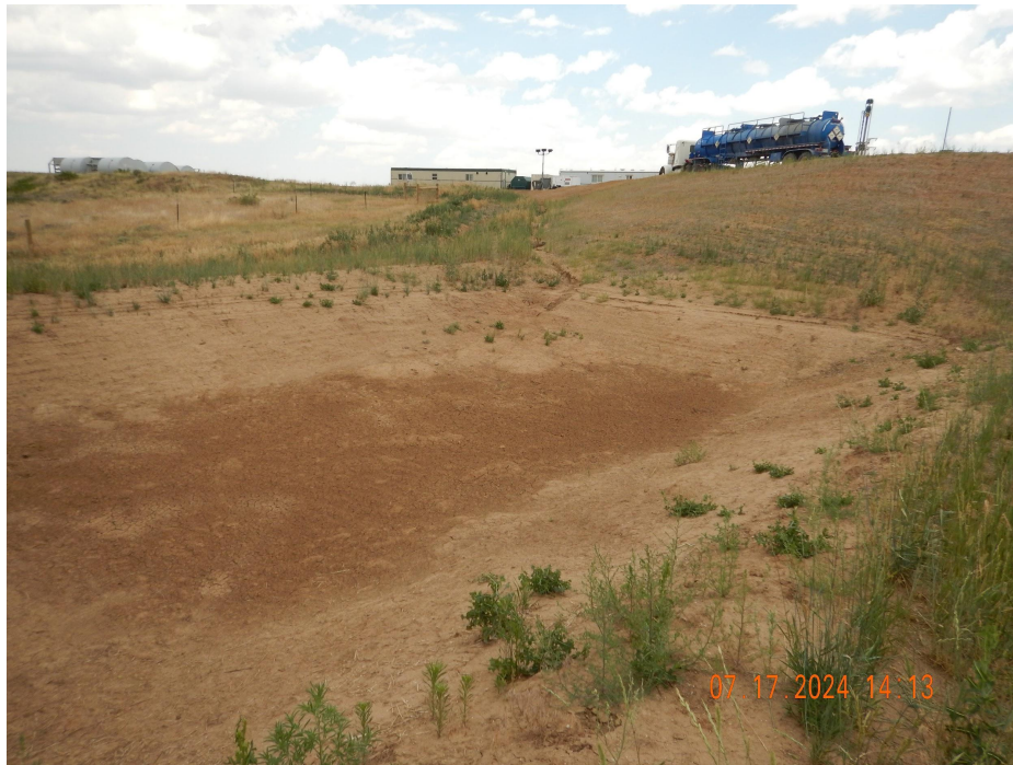
Photo 5. Photo taken along the western perimeter of location, facing Northeast. Photo illustrates some rill erosion coming into the inlet area.
