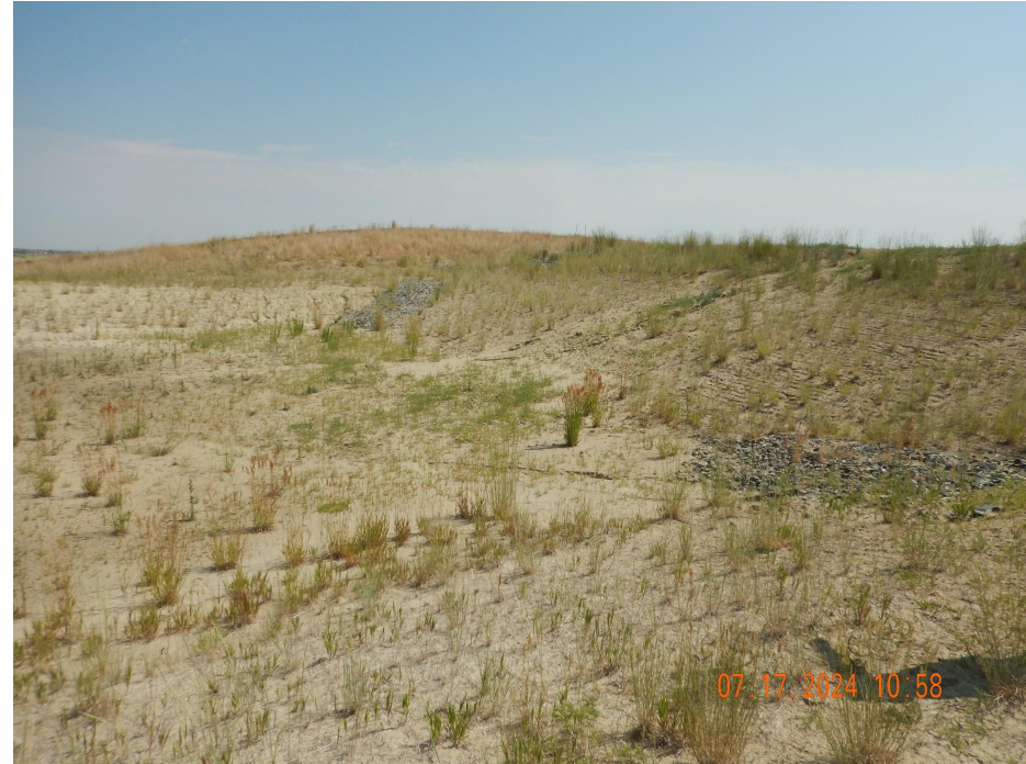
Photo 6. Photo taken along the northwestern perimeter of location, facing North. Some rill erosion was observed along the slopes of the retention pond.
