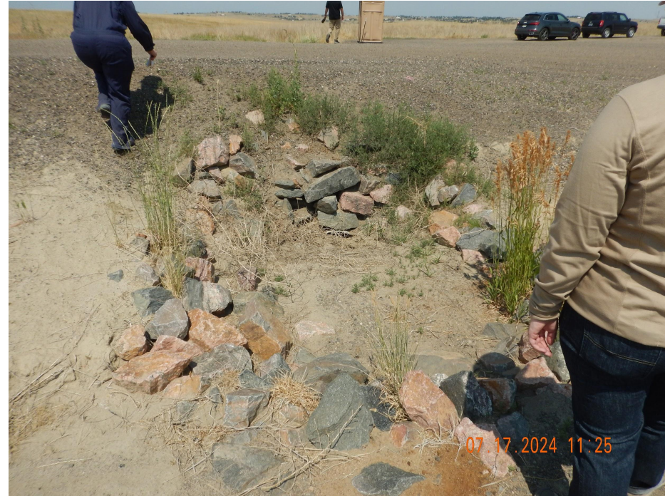
Photo 14. Photo taken along a portion of the access road west of the production facility, facing West. Photo illustrates a culvert in need of maintenance.
