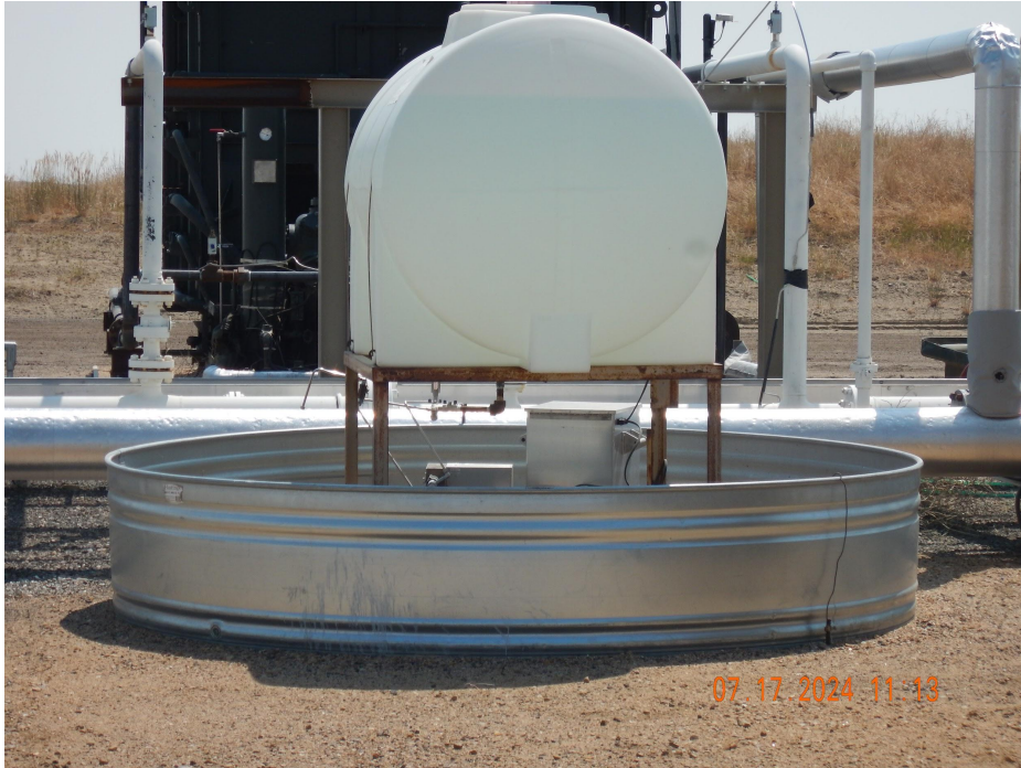
Photo 11. Photo taken along the southern production area, facing East. Photo illustrates wildlife protection devices (netting) are missing for secondary containment BMPs.
