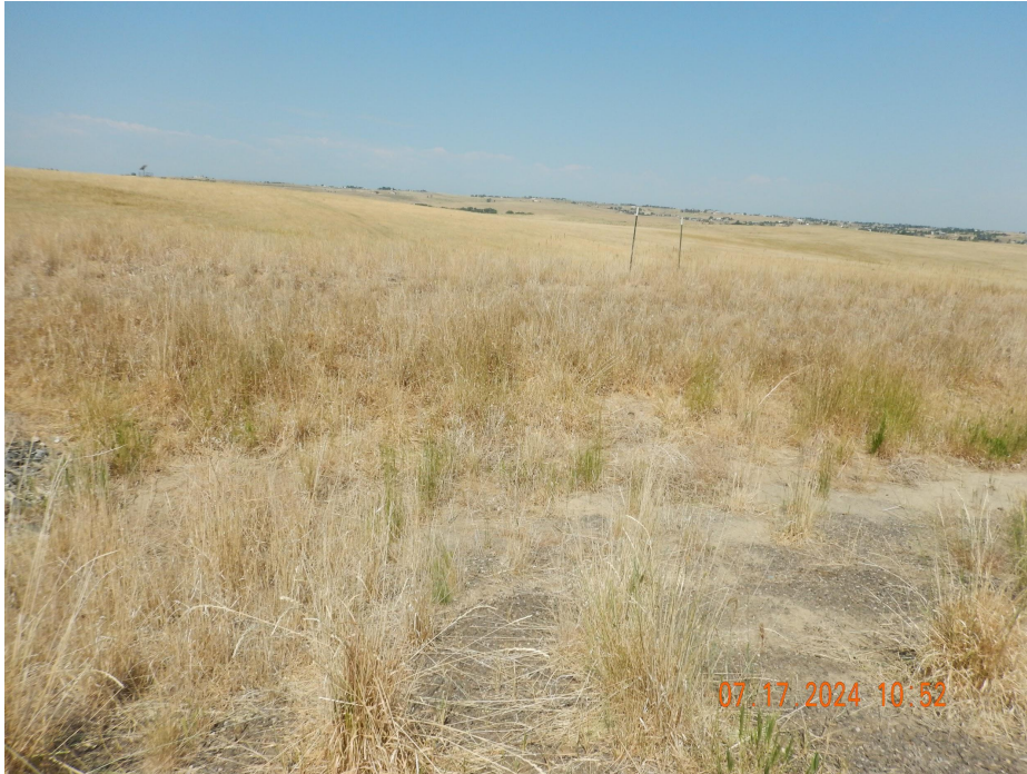
Photo 3. Photo taken along the western working pad surface, facing West. Photo illustrates the topsoil stockpile has been stabilized with an hybrid introduced/native grass mix.
