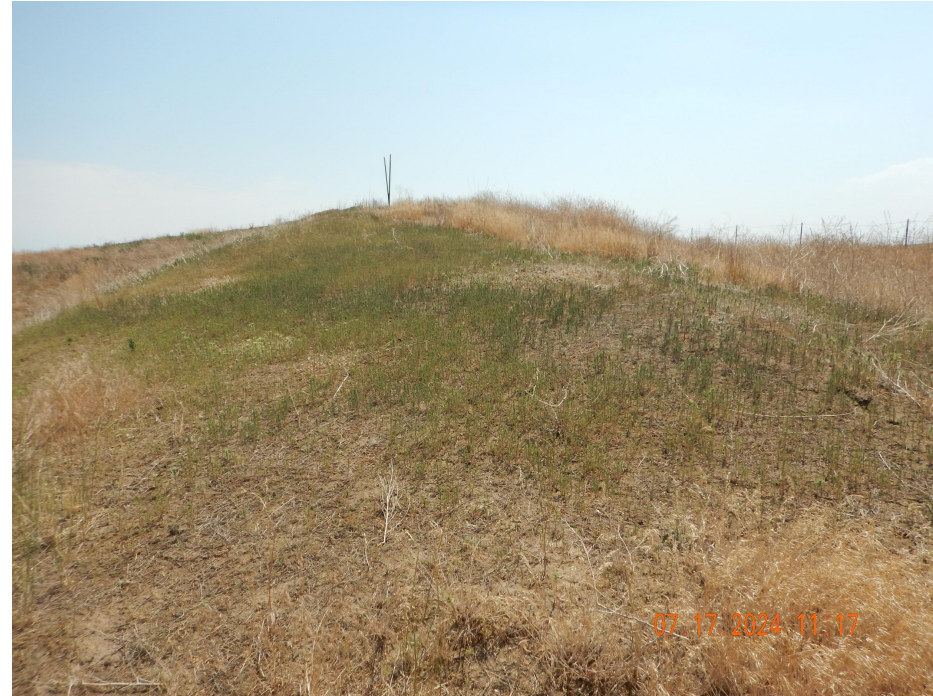
Photo 12. Photo taken along the southeastern perimeter of location, facing East. Photo illustrates the reclamation construction area is in process of vegetation establishment; however, there is a lack of desirable vegetation.
