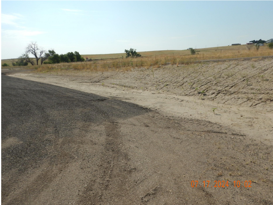
Photo 5. Photo taken along the southwestern working pad surface, facing Southeast. Photo illustrates rill erosion along the cut slope and sediment accumulation along the toe of the slope.
