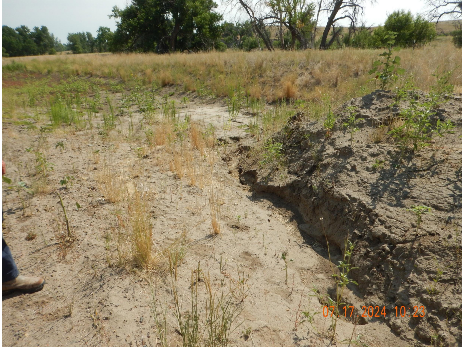
Photo 11. Photo taken from the eastern working pad surface, facing Northeast. Photo illustrates erosion into the retention pond.
