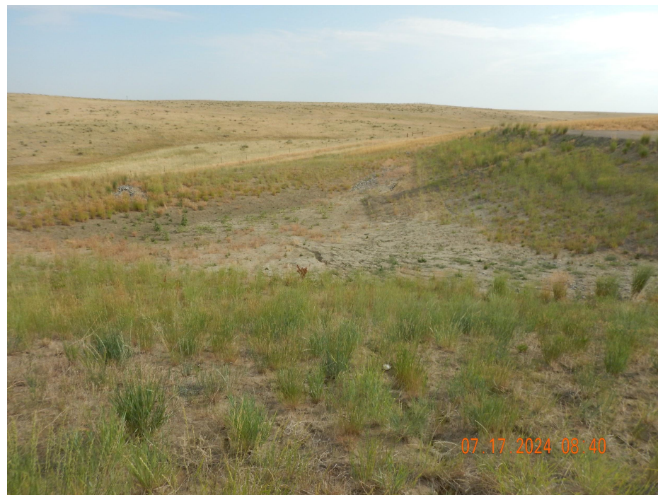
Photo 2. Photo taken along the northwestern working pad surface, facing Northwest. Photo illustrates a retention pond with a stabilized outlet.
