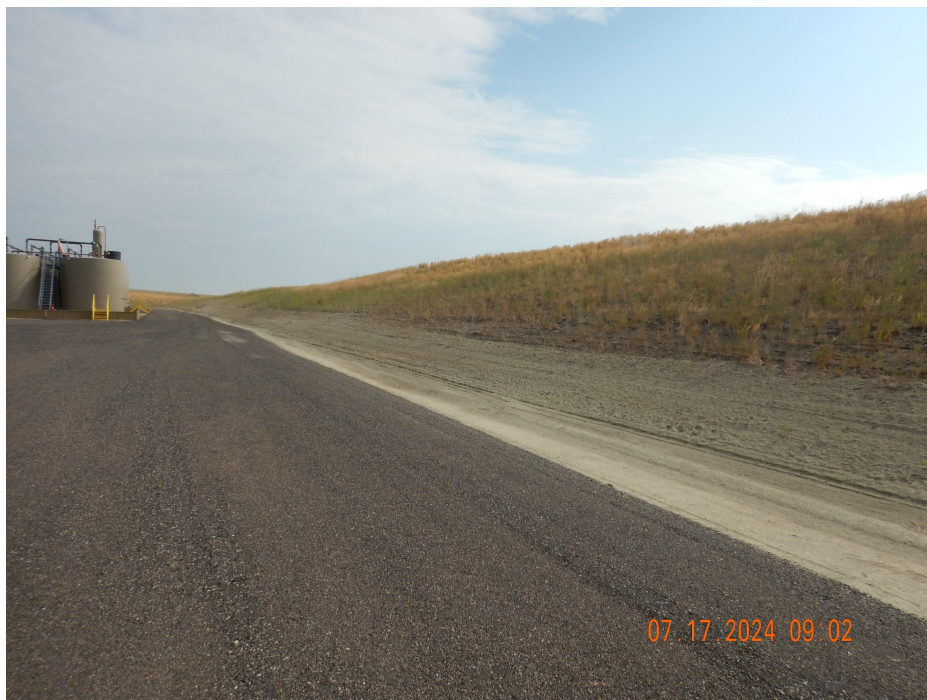
Photo 7. Photo taken from the eastern working pad surface, facing Northeast. Photo illustrates a portion of a cut slope that would require additional stabilization. Operator indicated stormwater repairs were conducted along the toe of the slope.
