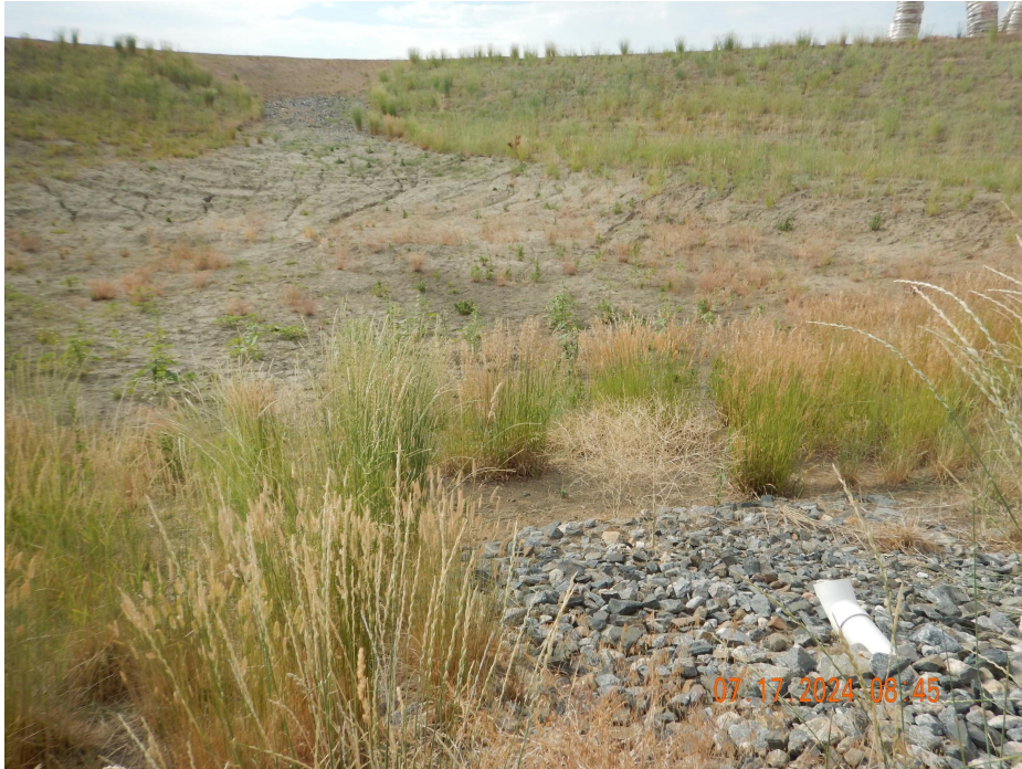
Photo 3. Close up photo taken from the stabilized outlet, facing Southeast. Photo illustrates rill erosion along the banks of the retention pond.
