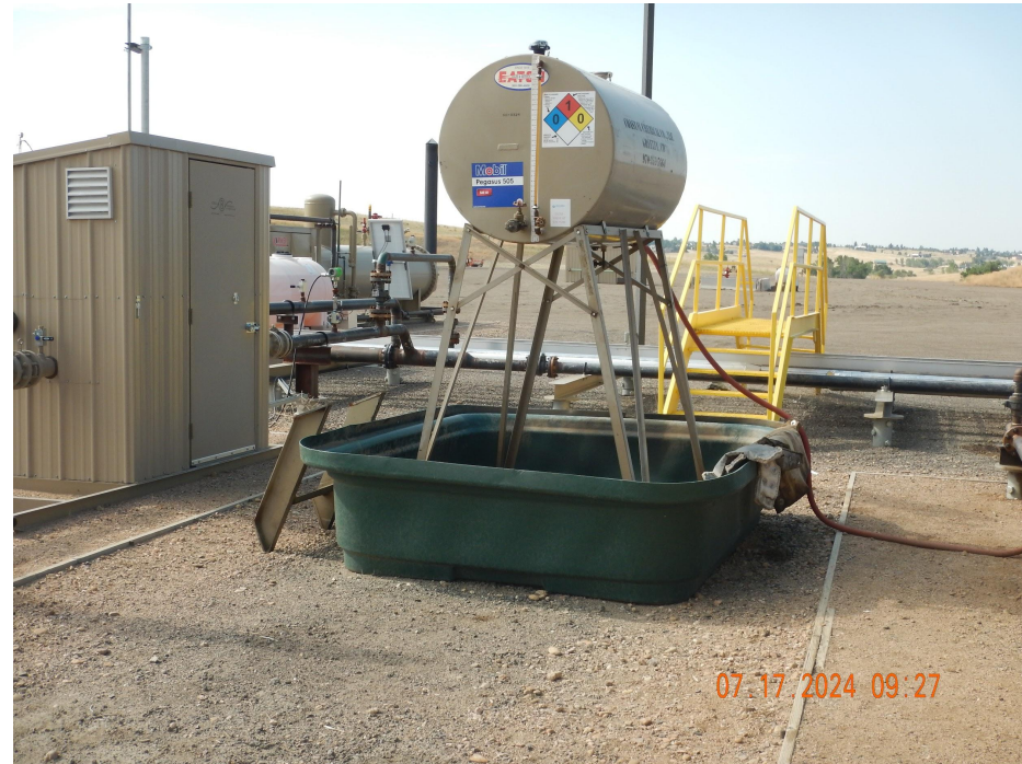
Photo 12. Photo taken from the northern production area illustrating the secondary containment lacks wildlife protection. Note- there was no observed fluids within the secondary containment at the time of this inspection.
