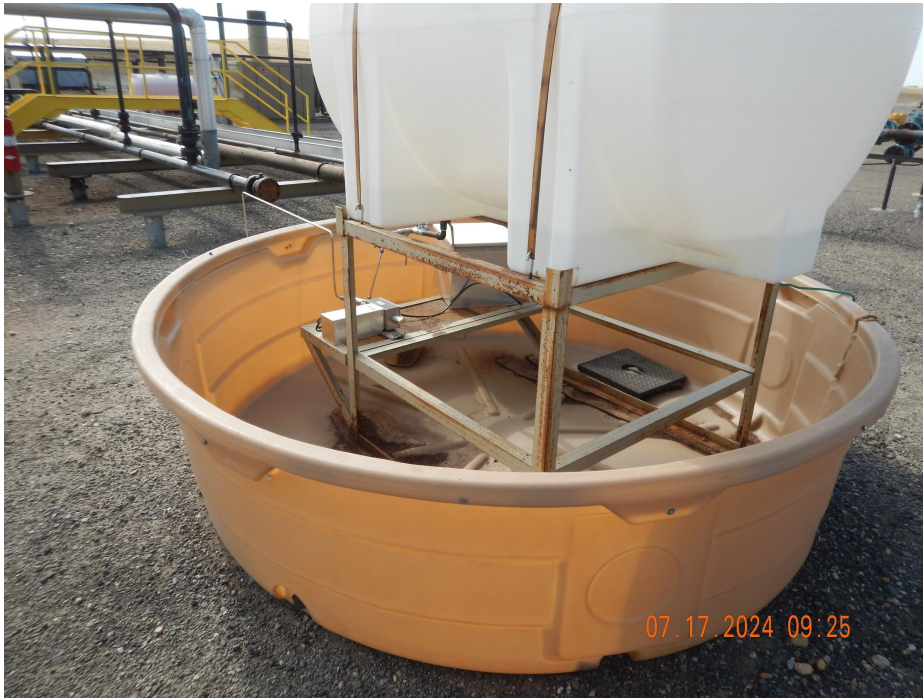
Photo 11. Photo taken from the northern production area illustrating the secondary containment lacks wildlife protection.
