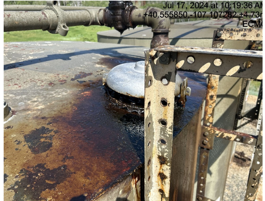
Thief hatch leaking
