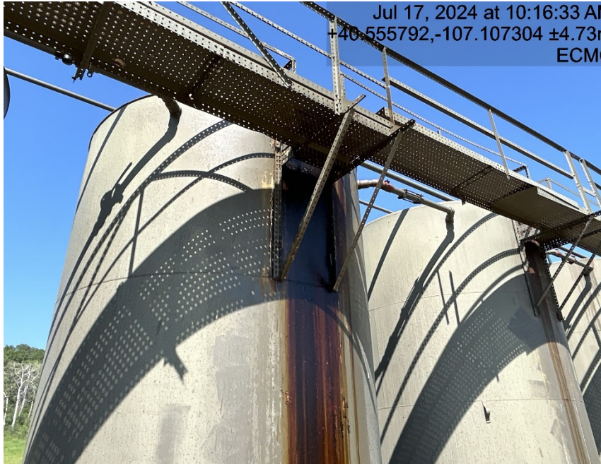
Staining down tank
