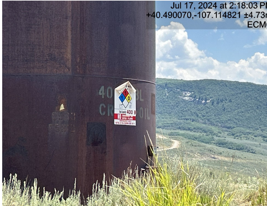
Tank labeling falling off
