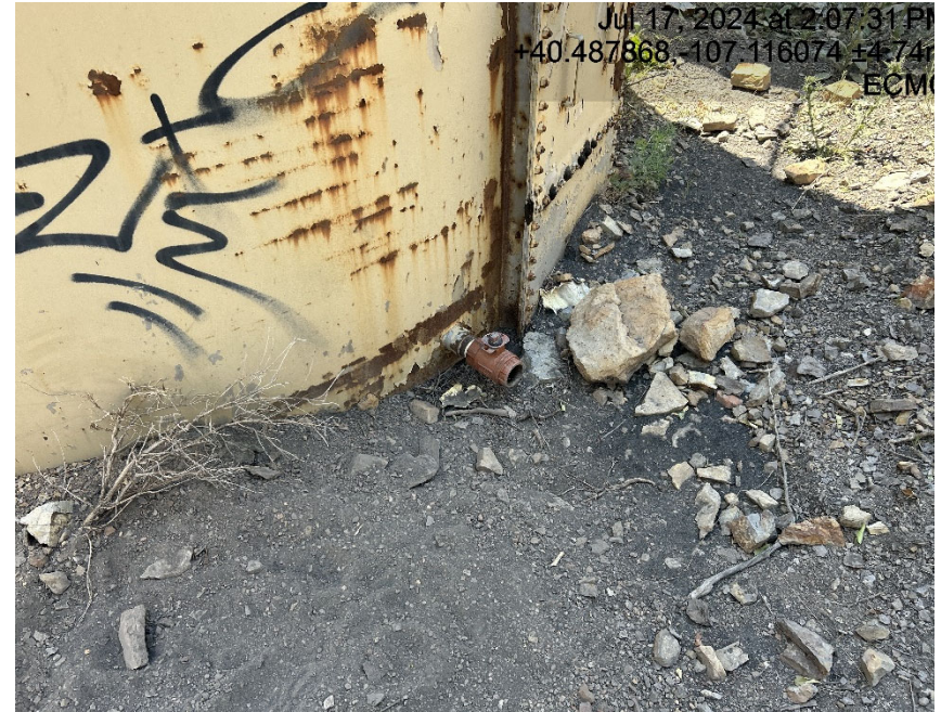
Load line missing cap/plug
