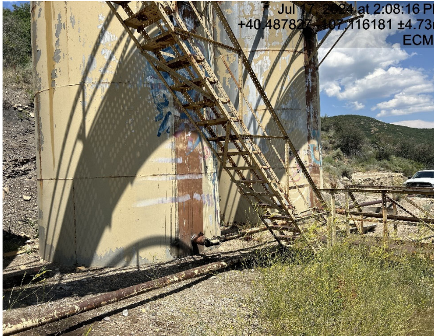
2 tanks missing labeling
