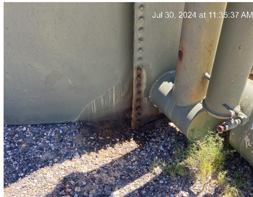
Hatch leaking and stained soil
