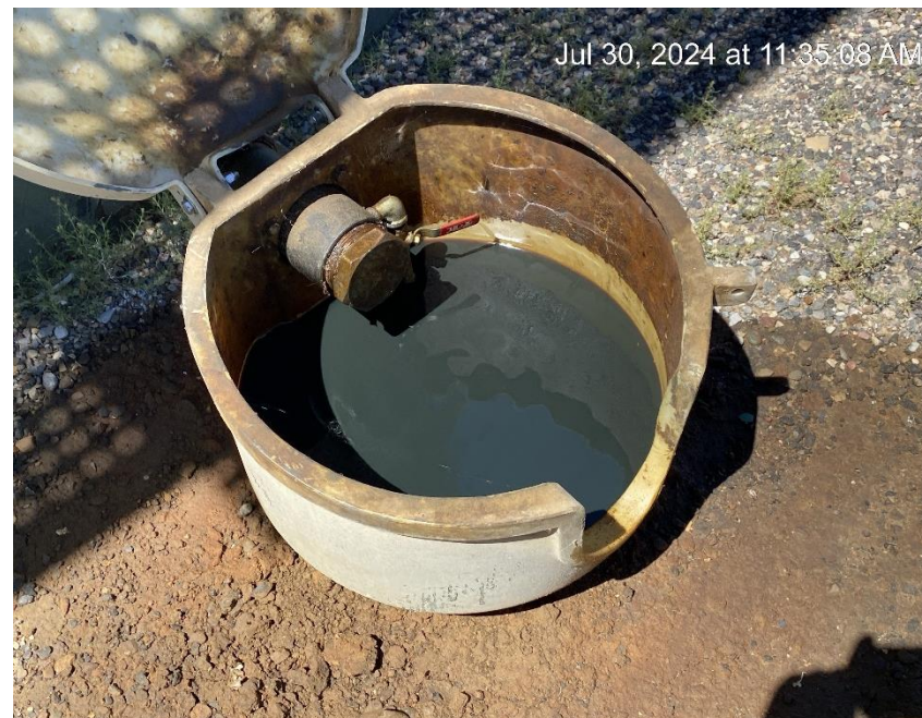
Loadout pot full of oil
