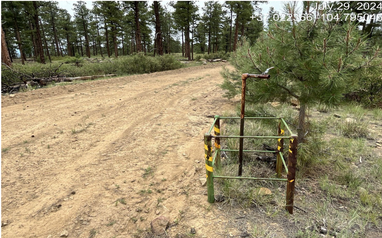
Photo 3. Further along the road another gas line with valve has no plug or lock to prevent accidental opening.
