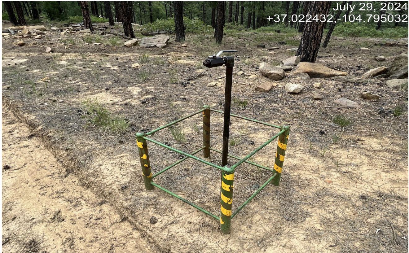
Photo 2. The gas line is closed and has a plug in it.
