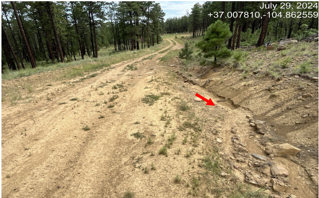
Photo 1. Facing northeast along the access road. There is erosion along the roadside which needs BMP's to control erosion. Tip: Rocks could be utilized to create check dam structures for erosion control.
