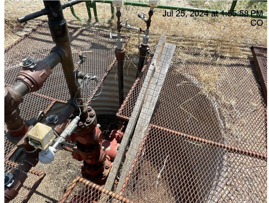
Photo # 3420 Wildlife egress damaged/needs maintenance
