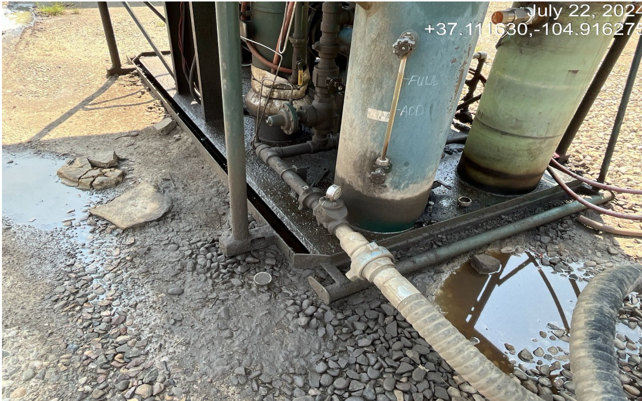
Photo 3. There is oil in the engine skid that has spilled over onto the ground and has mixed with stormwater..
