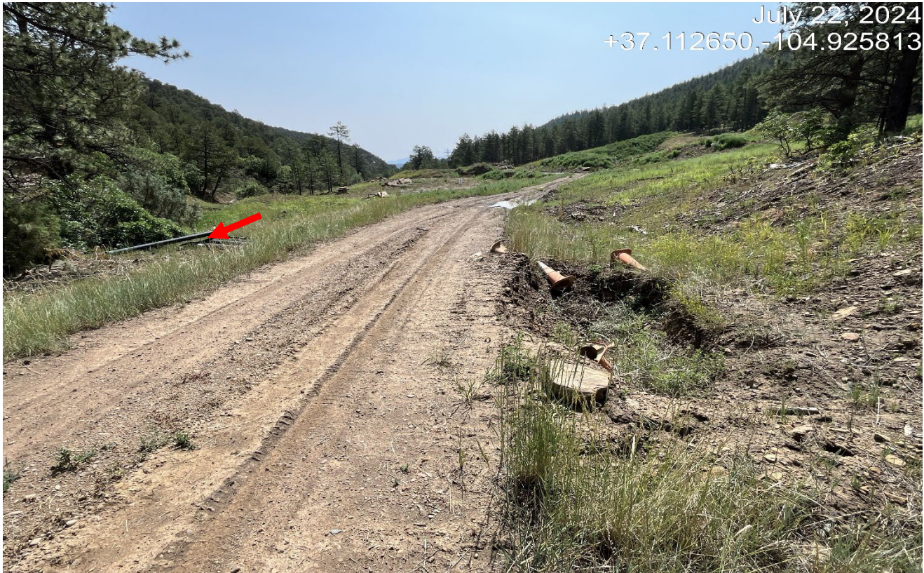
Photo 1. Facing west along the access road There are orange cones that have fallen over around this open hole. The open hole should be closed. There is also unused pipe at red arrow that needs to be removed.
