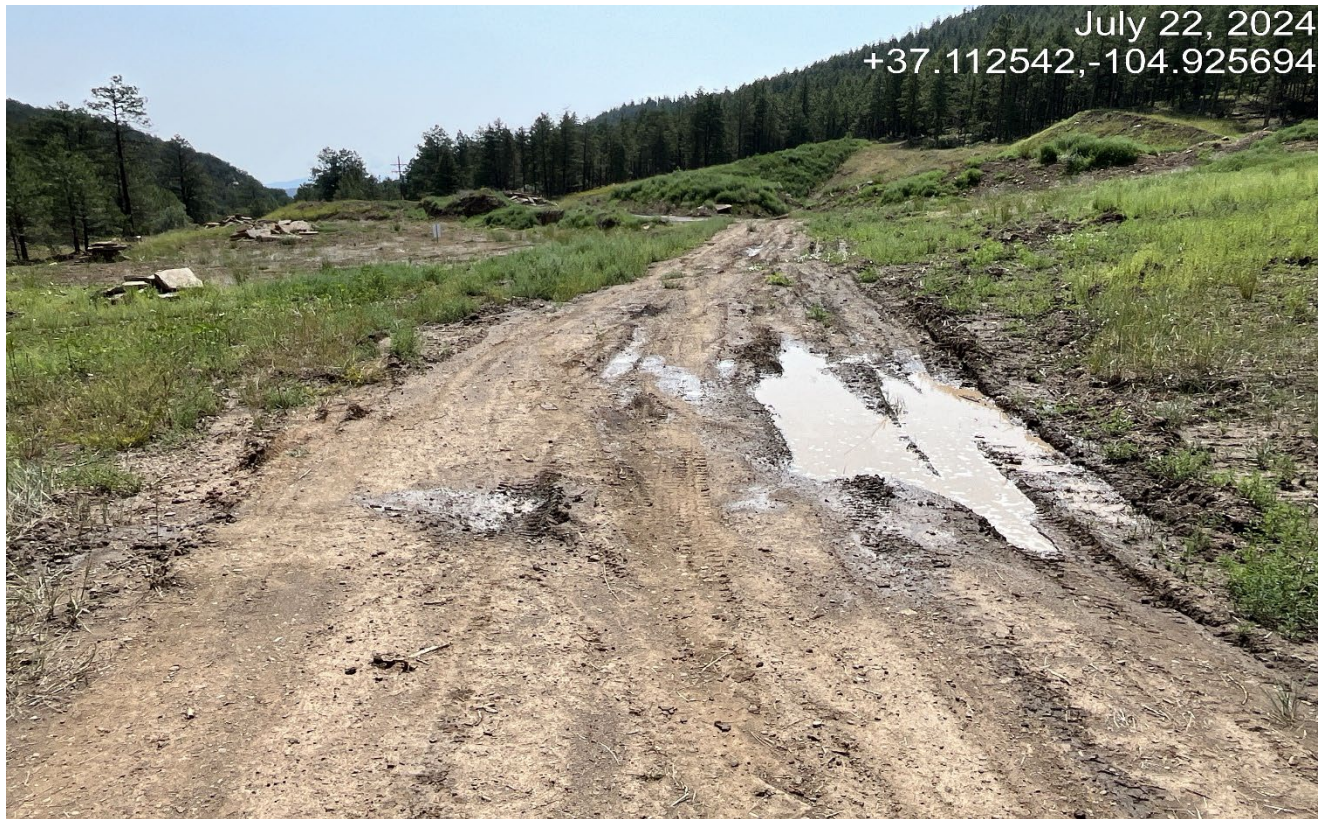
Photo 2. The access road thru the location needs to be maintained and stabilized with BMP's such as gravel.
