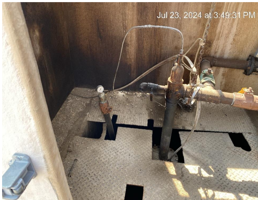
Production casing. No Bradenhead access
