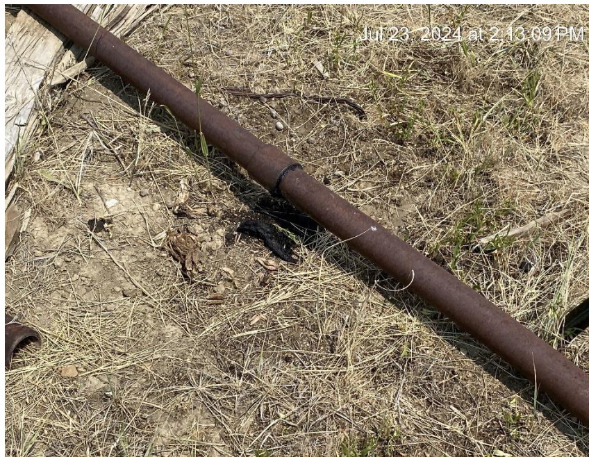
Flow line leak
