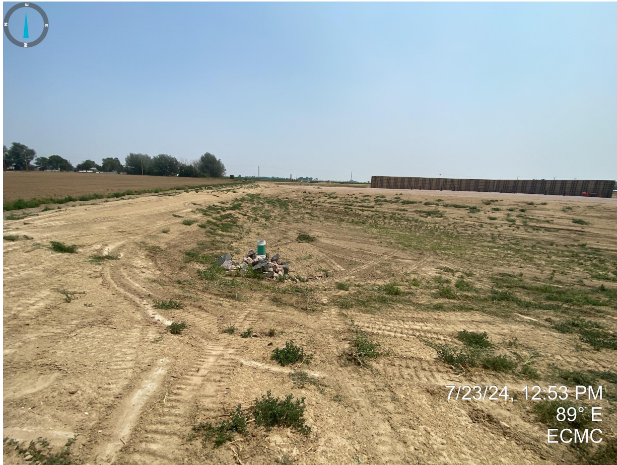
Photo 8. Northwest corner of the location, near the stormwater detention area. Undesirable vegetation appears to have recently been mowed or sprayed with herbicide. Equipment tracks on the hydromulch appear to have disturbed the application; no germination of desirable species observed at the time of this inspection.
