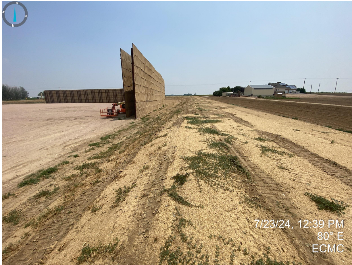
Photo 5. Southern portion of the topsoil stockpile. Equipment tracks on the hydromulch appear to have disturbed the application; no germination of desirable species observed at the time of this inspection.
