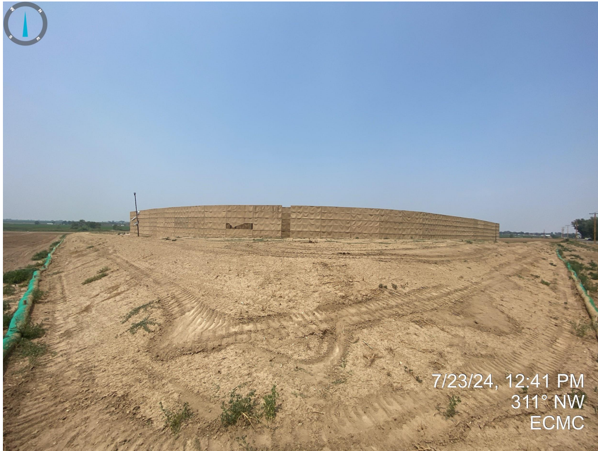
Photo 6. Southeast corner of the construction area. Photo illustrates a portion of the topsoil stockpile and perimeter control measures (e.g. filtrex wattles). Equipment tracks on the hydromulch appear to have disturbed the application; no germination of desirable species observed at the time of this inspection.
