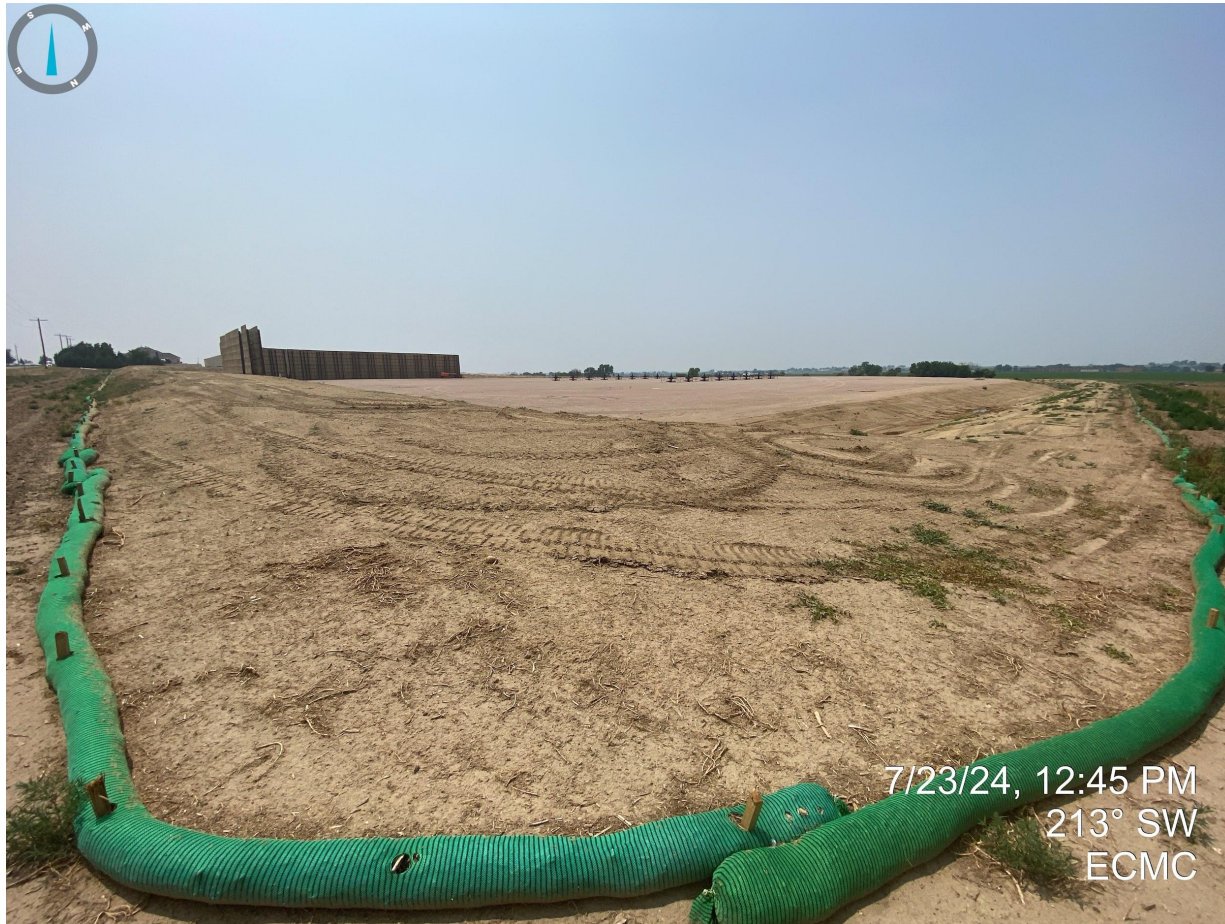
Photo 7. Northeast corner of the construction area. Photo illustrates a portion of the topsoil stockpile and perimeter control measures (e.g. filtrex wattles). Equipment tracks on the hydromulch appear to have disturbed the application; no germination of desirable species observed at the time of this inspection.
