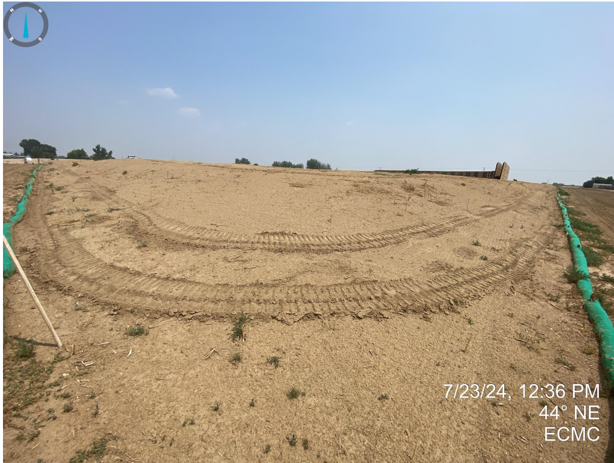
Photo 2. Southwest corner of the construction area. Photo illustrates a portion of the topsoil stockpile and perimeter control measures (e.g. filtrex wattles). Equipment tracks on the hydromulch appear to have disturbed the application; no germination of desirable species observed at the time of this inspection.
