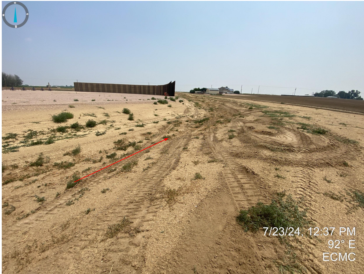
Photo 3. Southwest corner of the drilling pad. Photo illustrates stormwater ditch indicated by red arrow. Undesirable vegetation appears to have recently been mowed or sprayed with herbicide; equipment tracks on the hydromulch appear to have disturbed the application; no germination of desirable species observed at the time of this inspection.
