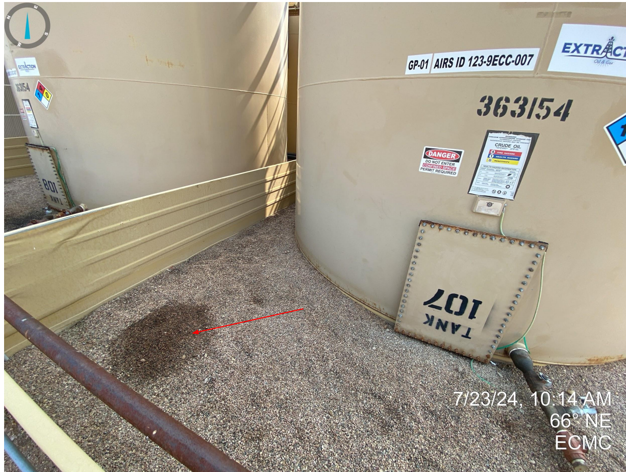
Photo 5. Stained soil within SW portion of tank battery.
