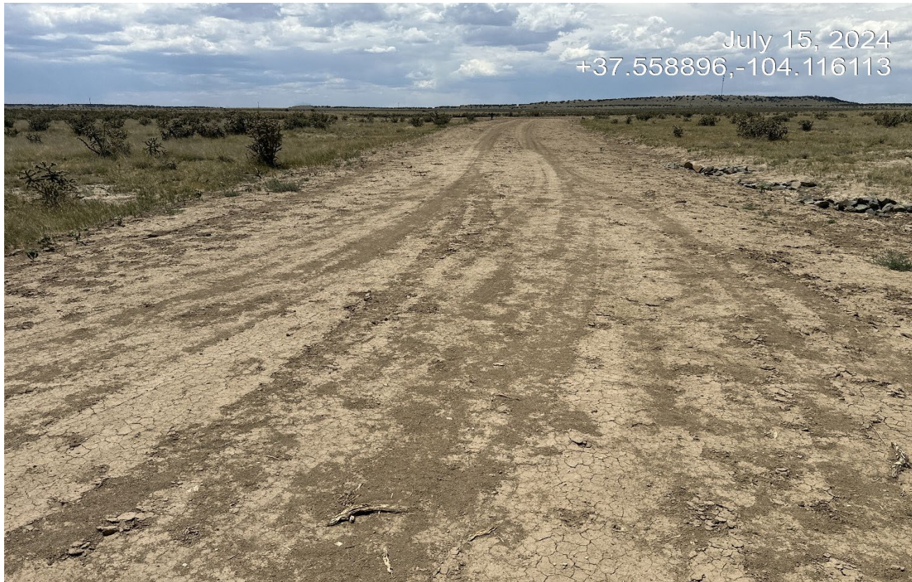
Photo 2. Facing northwest toward the access road. The side of the road needs to be seeded and stabilized
