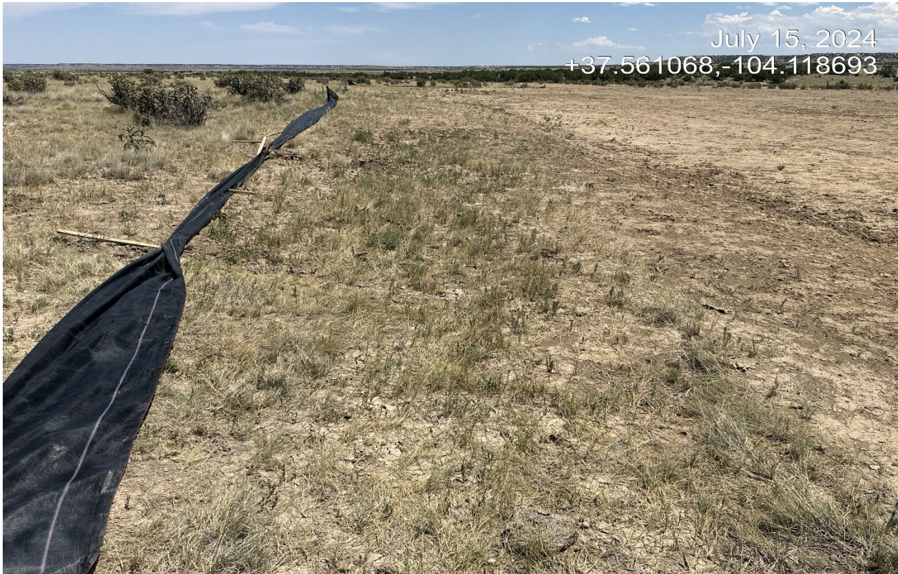
Photo 8. North side of the location facing east. The silt fence is down and not maintained.
