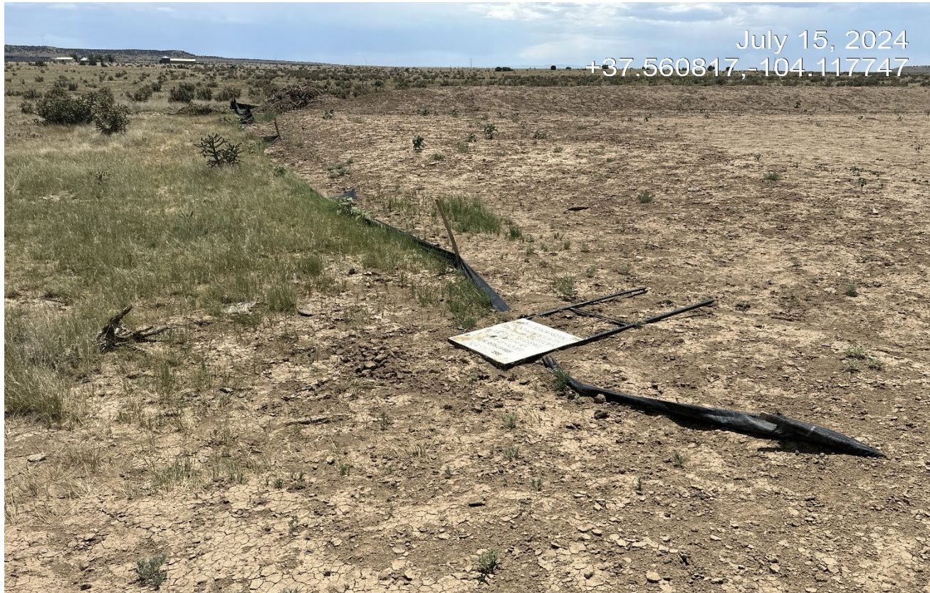
Photo 4. The sign has fallen over and the silt fence is down and not maintained.
