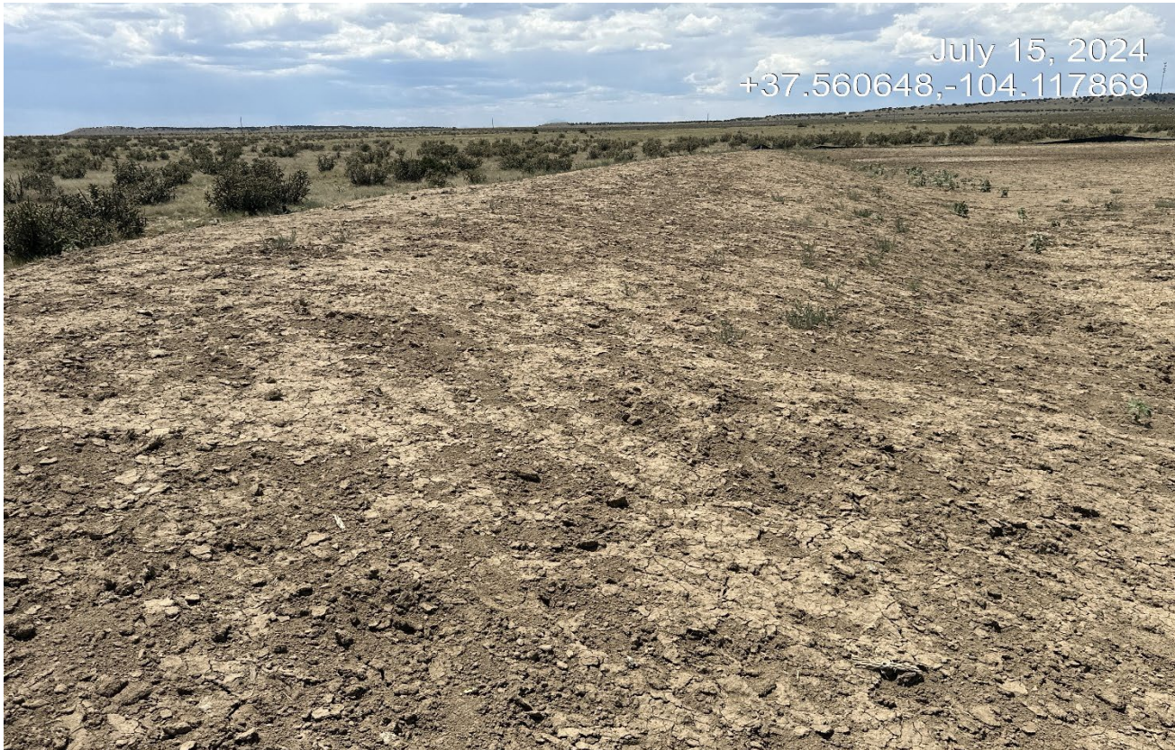
Photo 5. Facing toward the soil stock pile. The topsoil has not been seeded and stabilized and weeds are beginning to establish.
