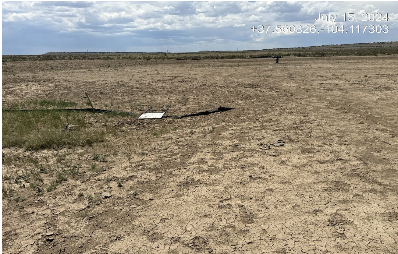
Photo 3. Facing northwest toward the location. The sign has fallen over and the silt fence is down and not maintained.
