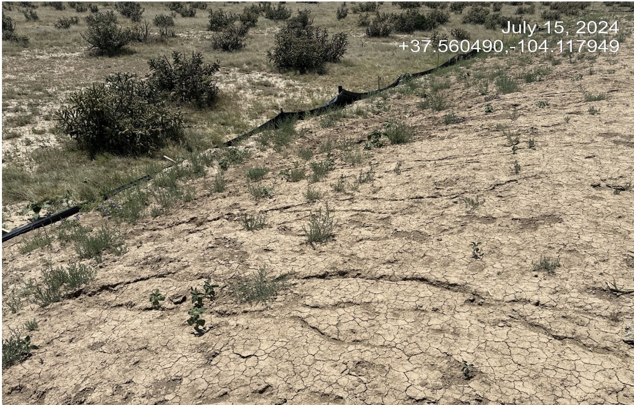
Photo 6. Facing toward the backside of the soil stock pile. There is erosion occurring along the topsoil pile and the silt fence is in disrepair.
