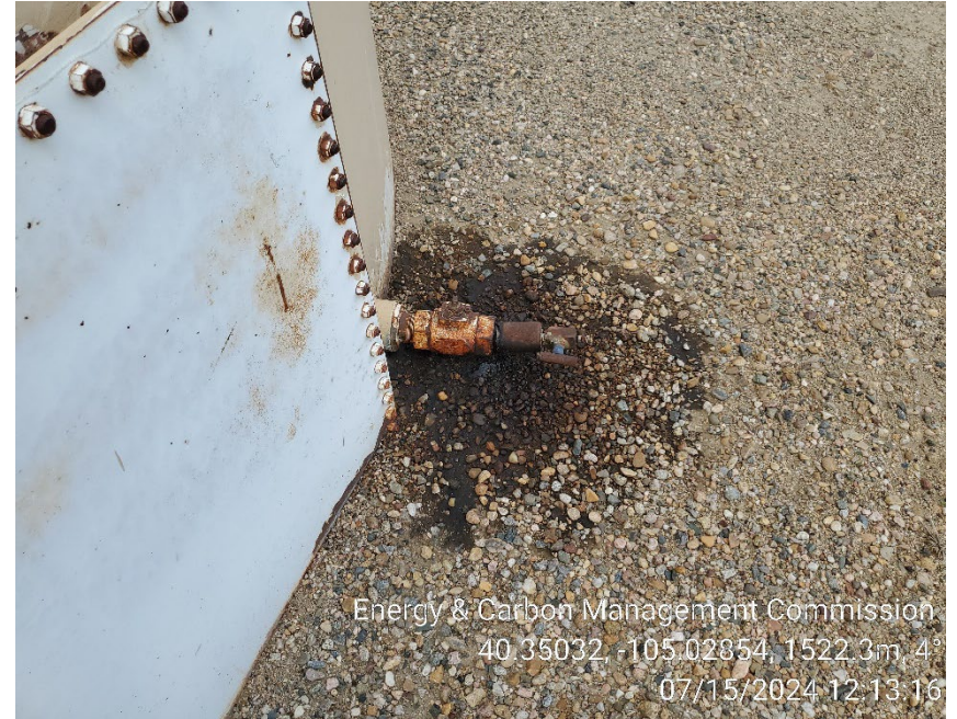
Crude oil tank drain valve and stained soil
