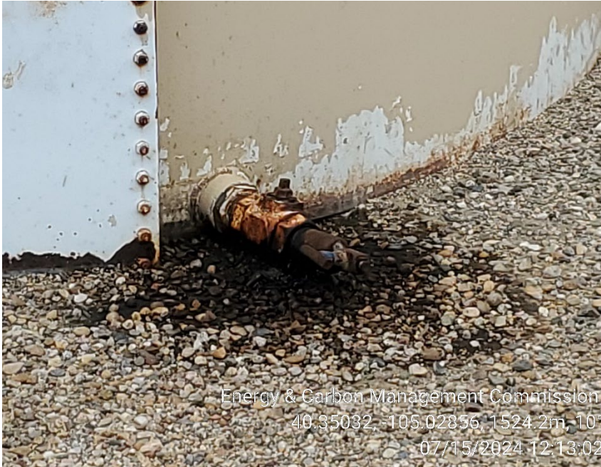
Crude oil tank drain valve and stained soil
