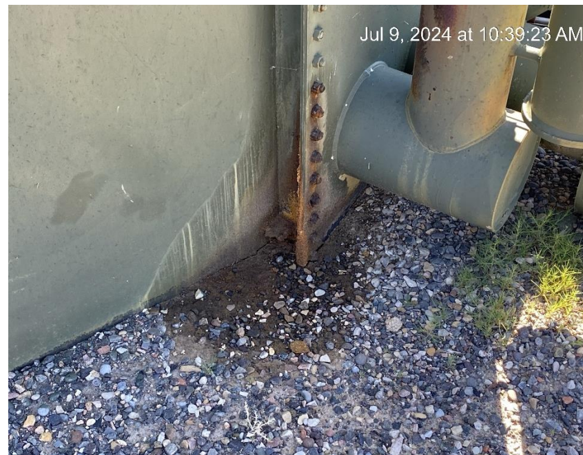
Leaking equipment. Stained soil.
