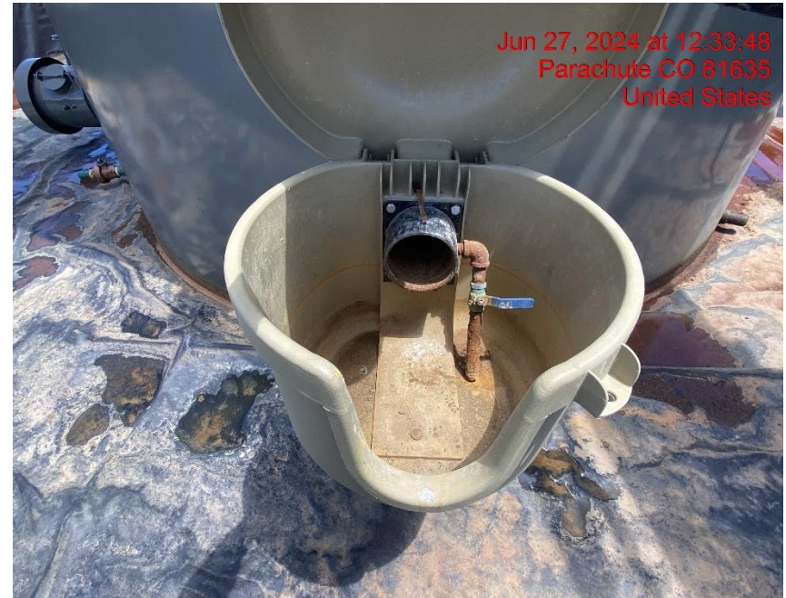
Open-Ended Load Line – Photo #02054
