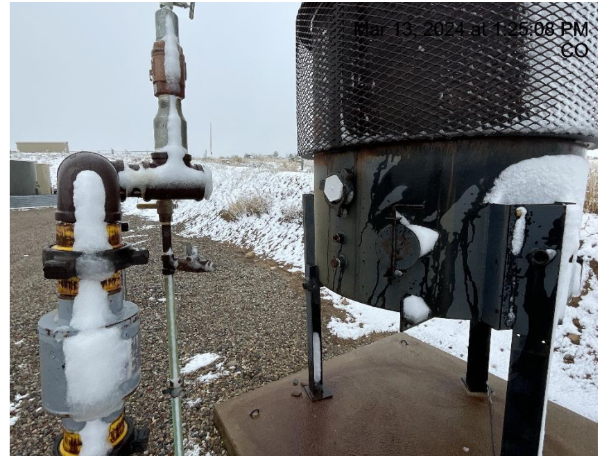
Photo # 9873 From inspection 708903328 conducted on 03/13/2024 Unused equipment/ECD disconnected
