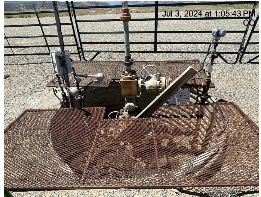
Photo # 2558 Cellar cover not properly installed/wildlife & personnel hazard & wildlife egress not properly installed.
