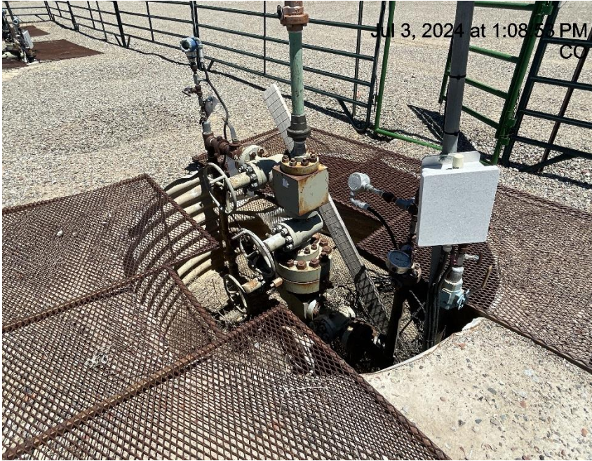
Photo # 2559 Cellar cover not properly installed/wildlife & personnel hazard & wildlife egress not properly installed.
