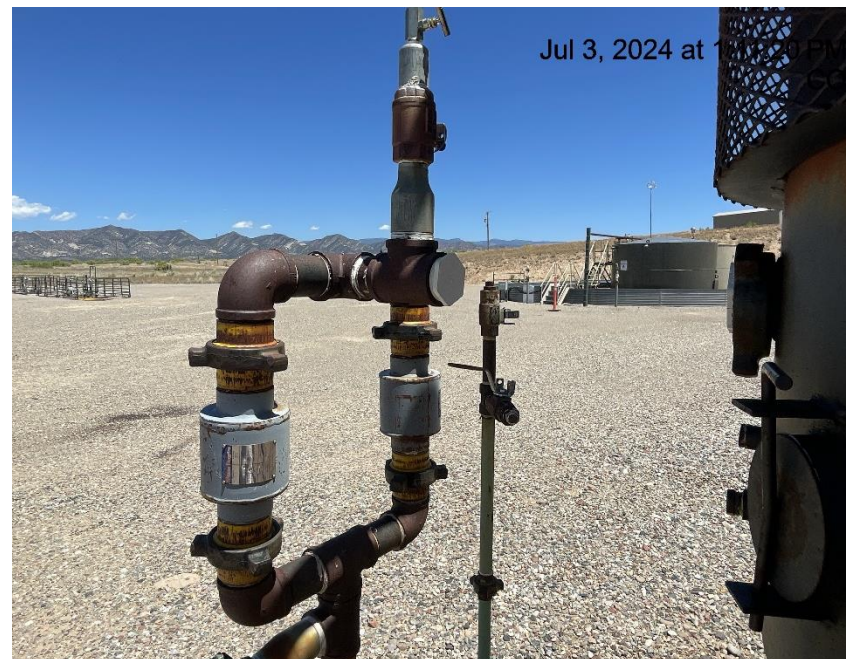
Photo # 2557 Unused equipment/ECD disconnected
