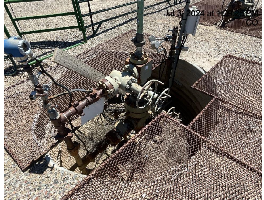
Photo # 2560 Cellar cover not properly installed/wildlife & personnel hazard & wildlife egress not properly installed.
