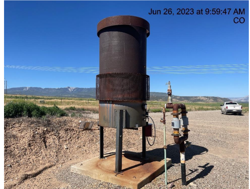
Photo # 1802 from inspection 708900877 conducted on 06/26/2023 - Unused equipment/ECD disconnected
