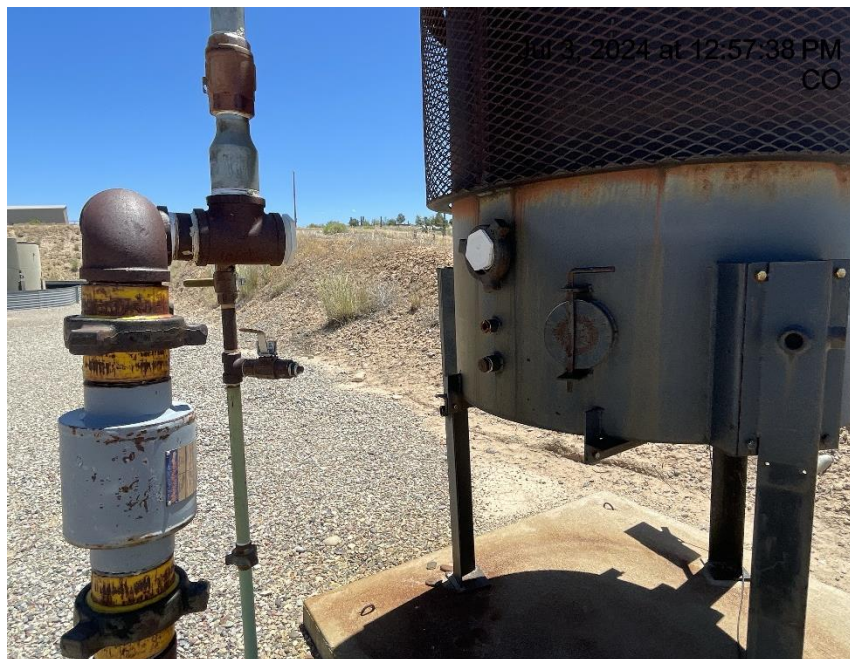
Photo # 2556 Unused equipment/ECD disconnected
