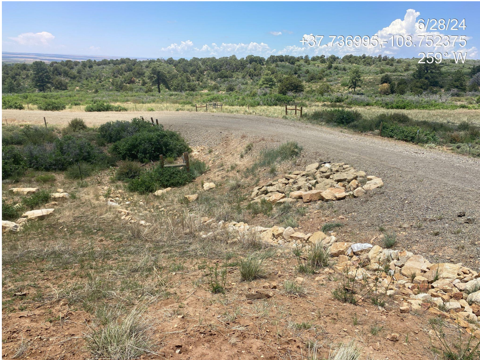
Photo 5. View of storm water BMPs that are functioning and have been properly maintained near the access point of the disturbance.
