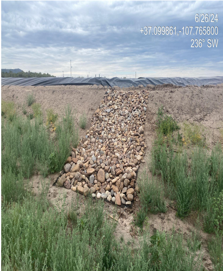
Photo 6. View of functioning and maintained storm water BMPs along the perimeter of the tank pad.
