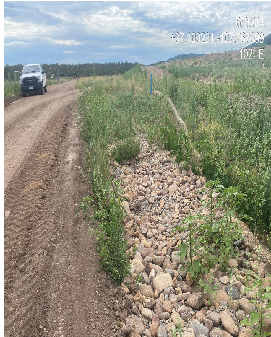
Photo 4. View of functioning and maintained storm water BMPs along existing access road separating the well and tank pads.
