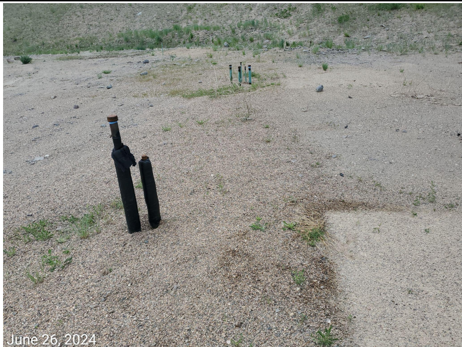
Photo 15: Photos examples showing unused riser equipment has not been removed from the Location.
