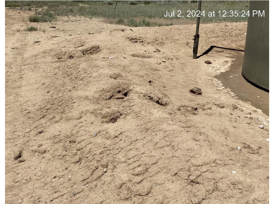
Inadequate tank containment
