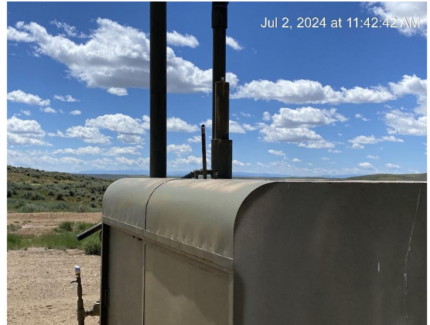
Relief riser cap missing
