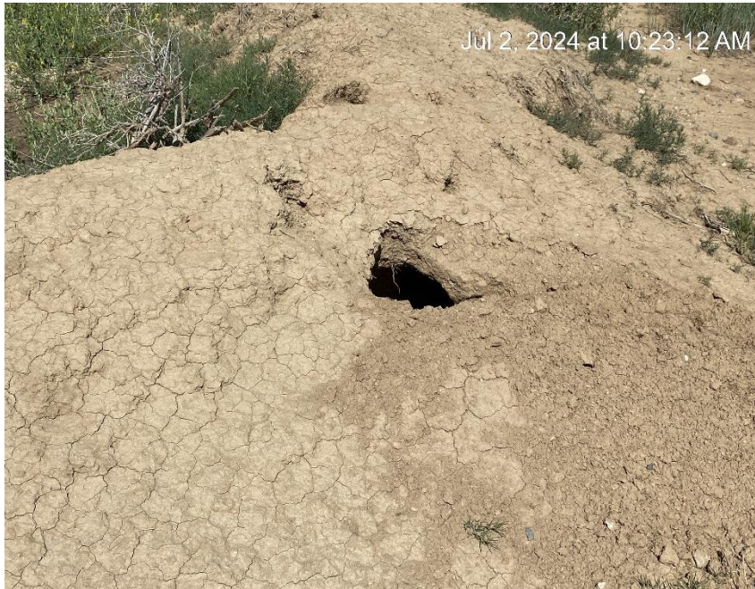
Inadequate tank berm
