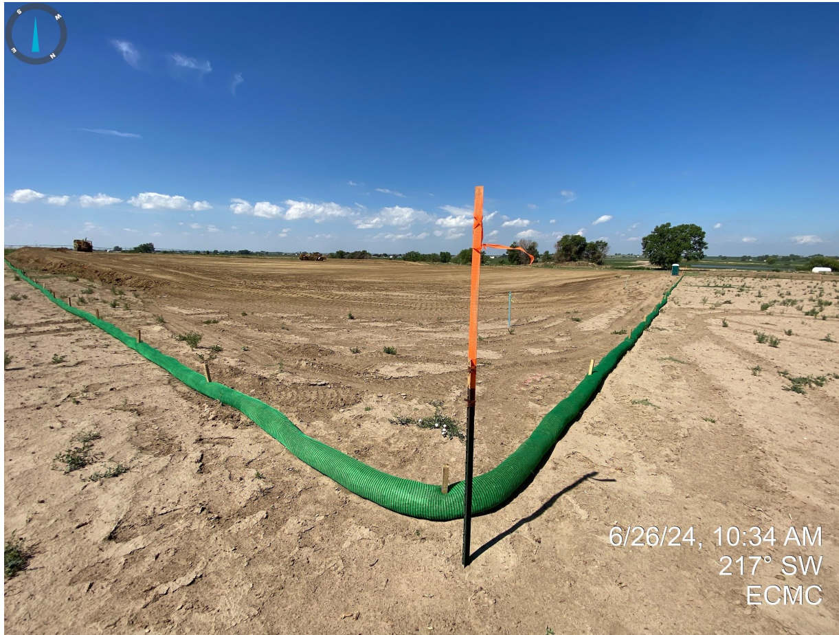
Photo 5. Northeast corner of the construction area. Temporary BMPs (filtrexx wattles) have been installed along the entire perimeter during the construction phase. More permanent BMPs should be selected and installed upon completion of the pad.
