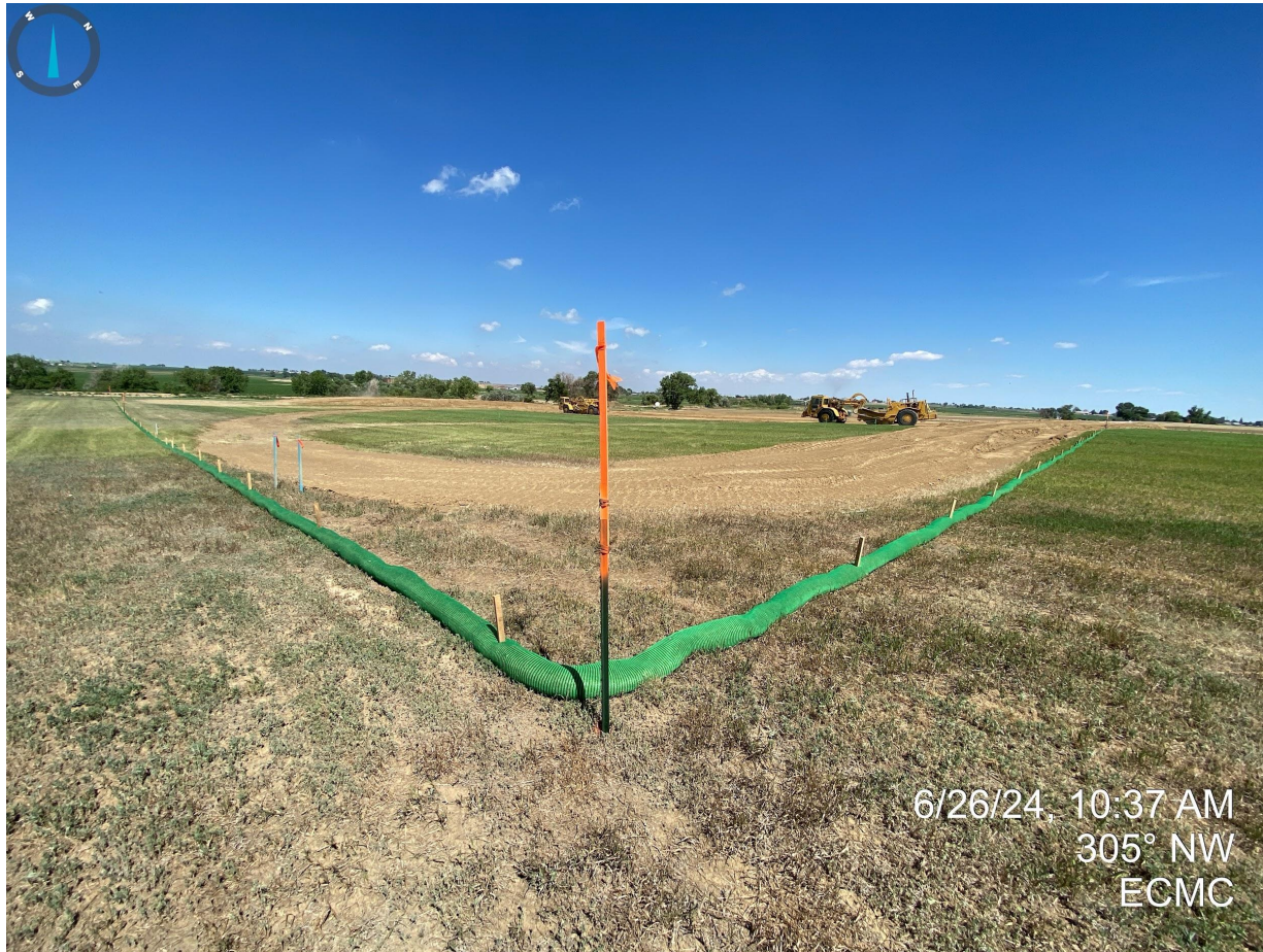
Photo 9. Southeast corner of the construction area. Temporary BMPs (filtrexx wattles) have been installed along the entire perimeter during the construction phase. More permanent BMPs should be selected and installed upon completion of the pad.
