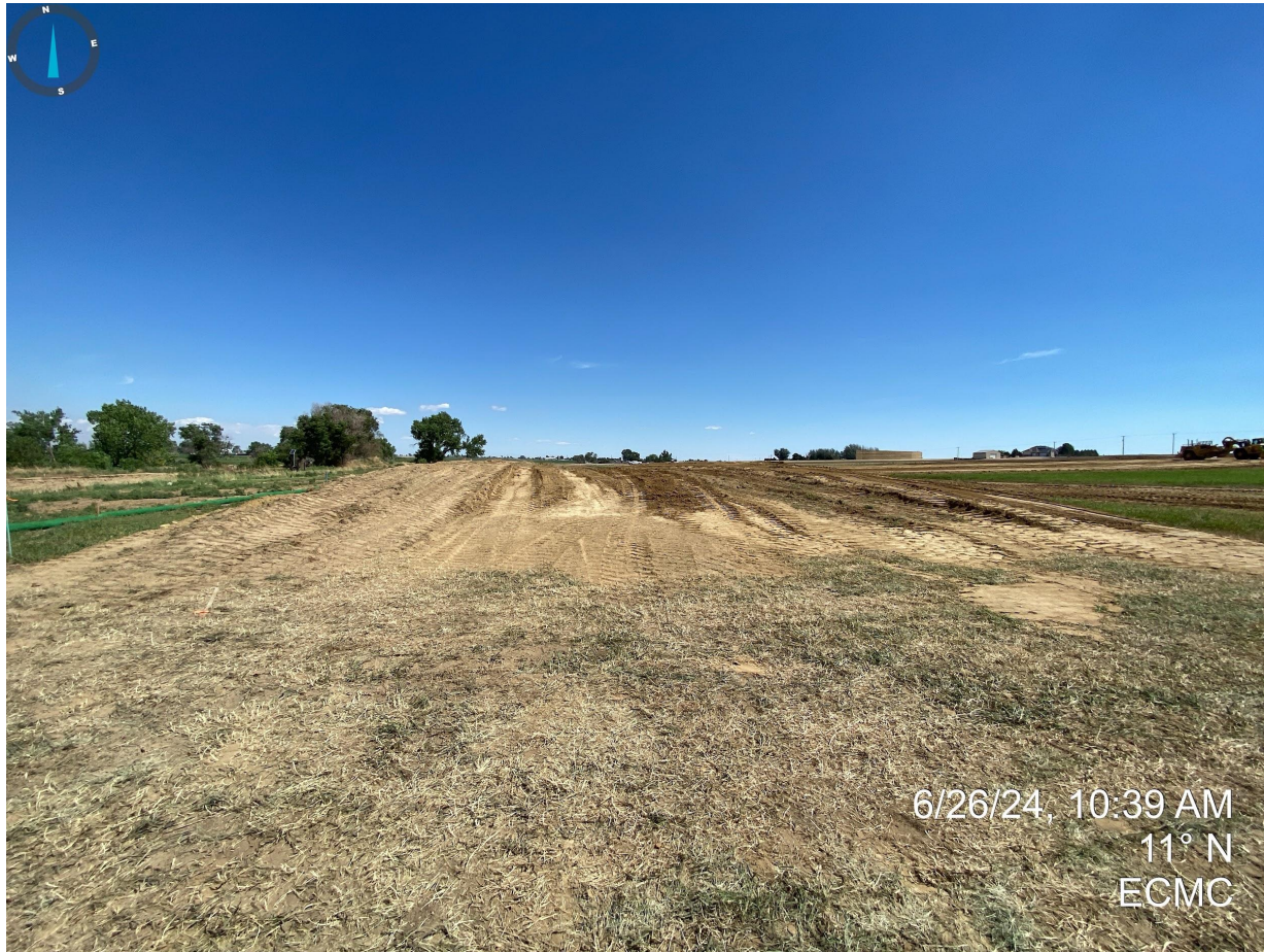
Photo 11. Topsoil stockpile on the western portion of the location. Topsoil salvage activities were ongoing at the time of this inspection.
