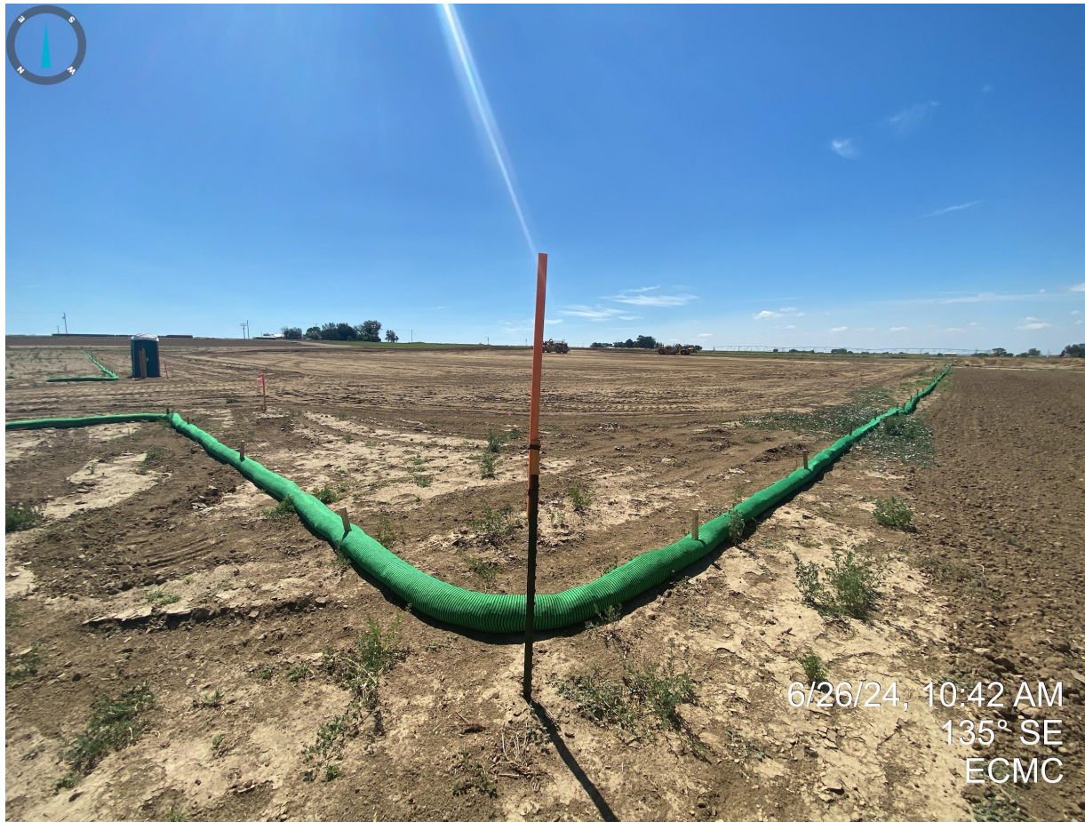
Photo 13. Northwest corner of the construction area. Temporary BMPs (filtrexx wattles) have been installed along the entire perimeter during the construction phase. More permanent BMPs should be selected and installed upon completion of the pad.
