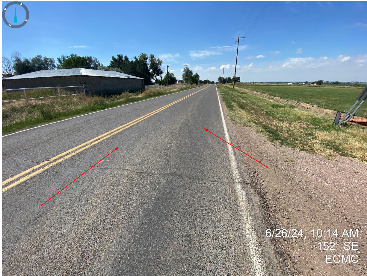
Photo 1. Facing south on WCR 51, near the location entrance. Vehicle track out observed originating from the location entrance.
