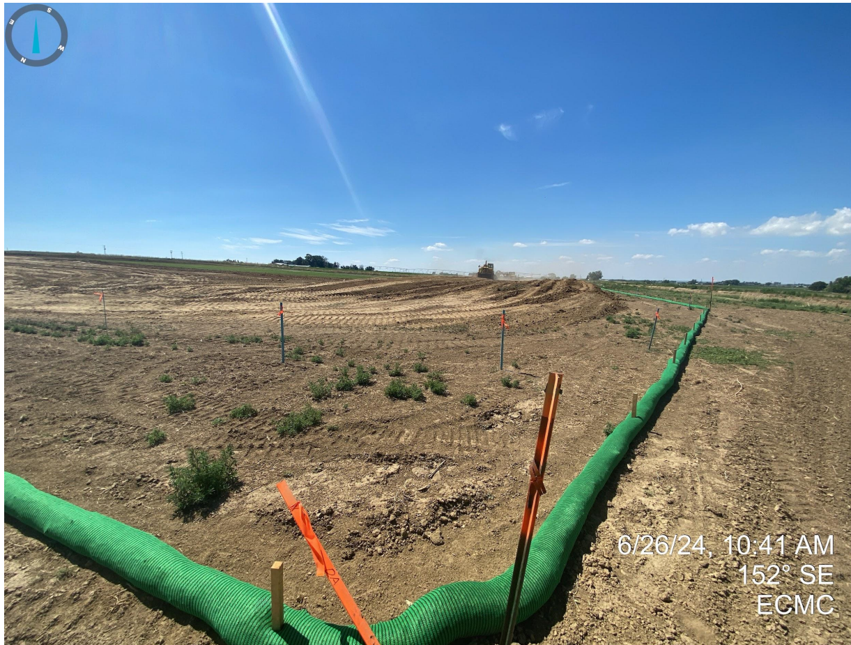
Photo 12. West/center portion of the construction area. Temporary BMPs (filtrex wattles) have been installed along the entire perimeter during the construction phase. More permanent BMPs should be selected and installed upon completion of the pad.
