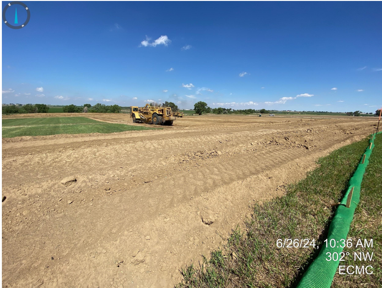
Photo 8. Topsoil salvage activities were ongoing at the time of this inspection. The Operator shall ensure that all topsoil is salvaged from the location, in compliance with Rule 1002.b.
