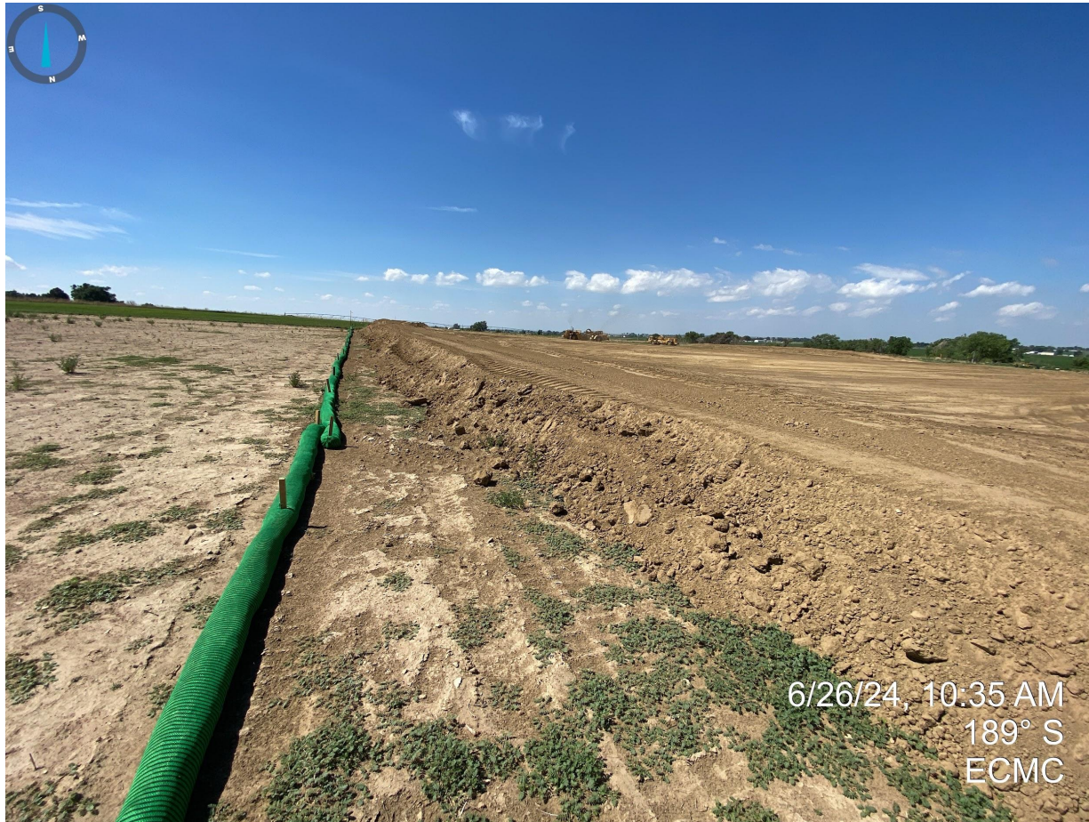
Photo 6. Topsoil stockpile on the eastern portion of the pad; topsoil salvage activities were ongoing at the time of this inspection.
