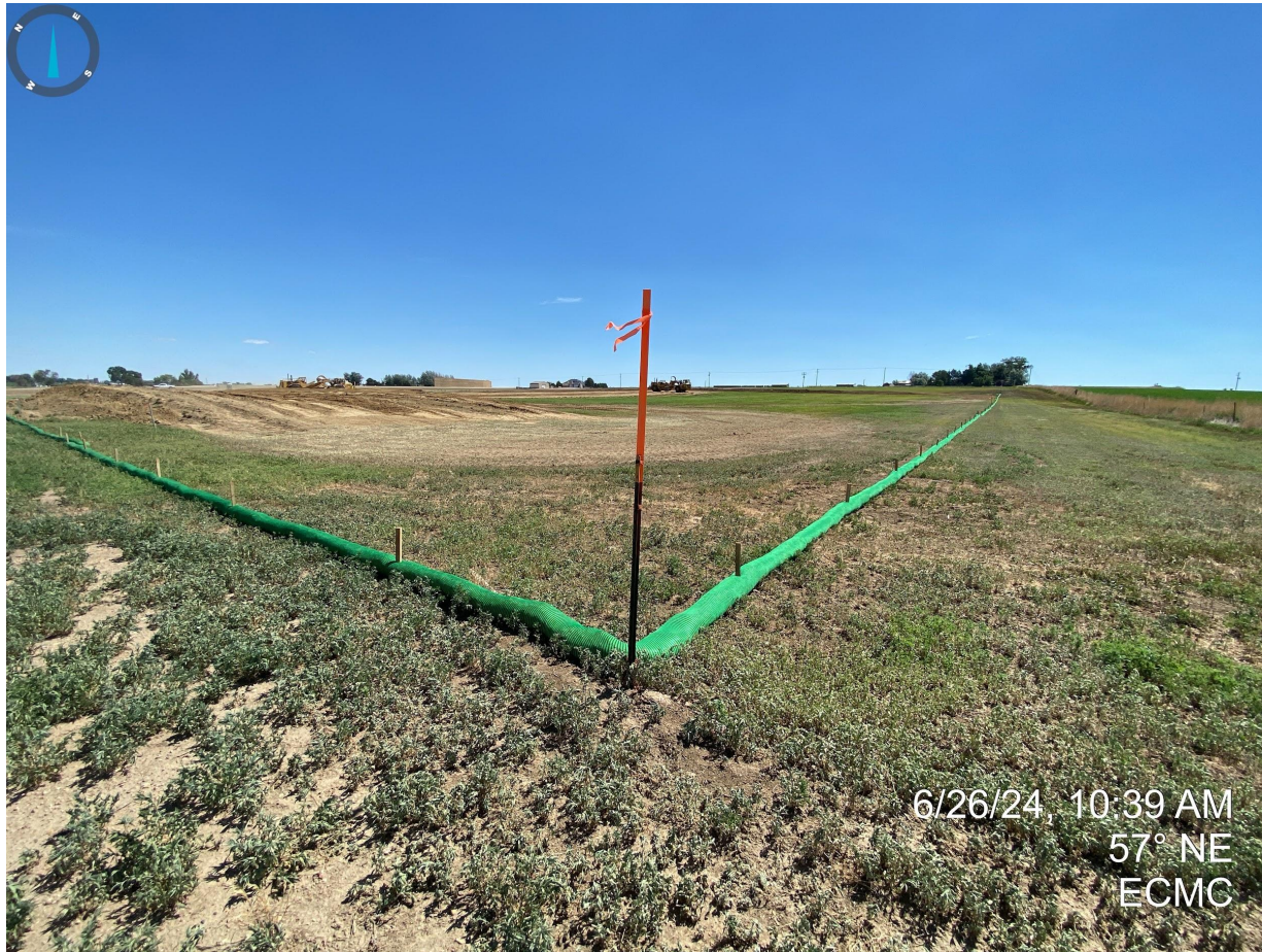
Photo 10. Southwest corner of the construction area. Temporary BMPs (filtrexx wattles) have been installed along the entire perimeter during the construction phase. More permanent BMPs should be selected and installed upon completion of the pad.
