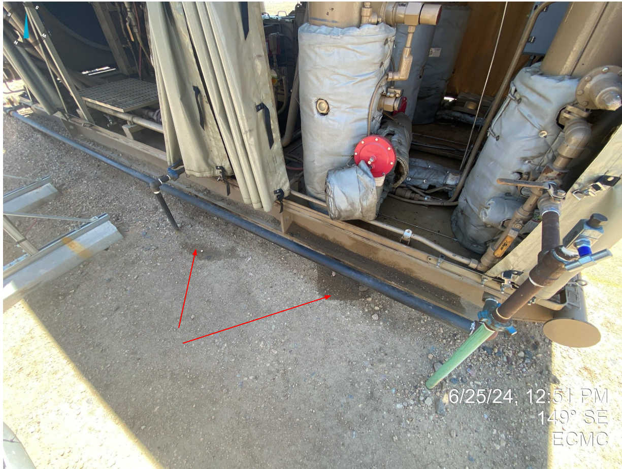
Photo 6. Stained soil at compressor skid.
