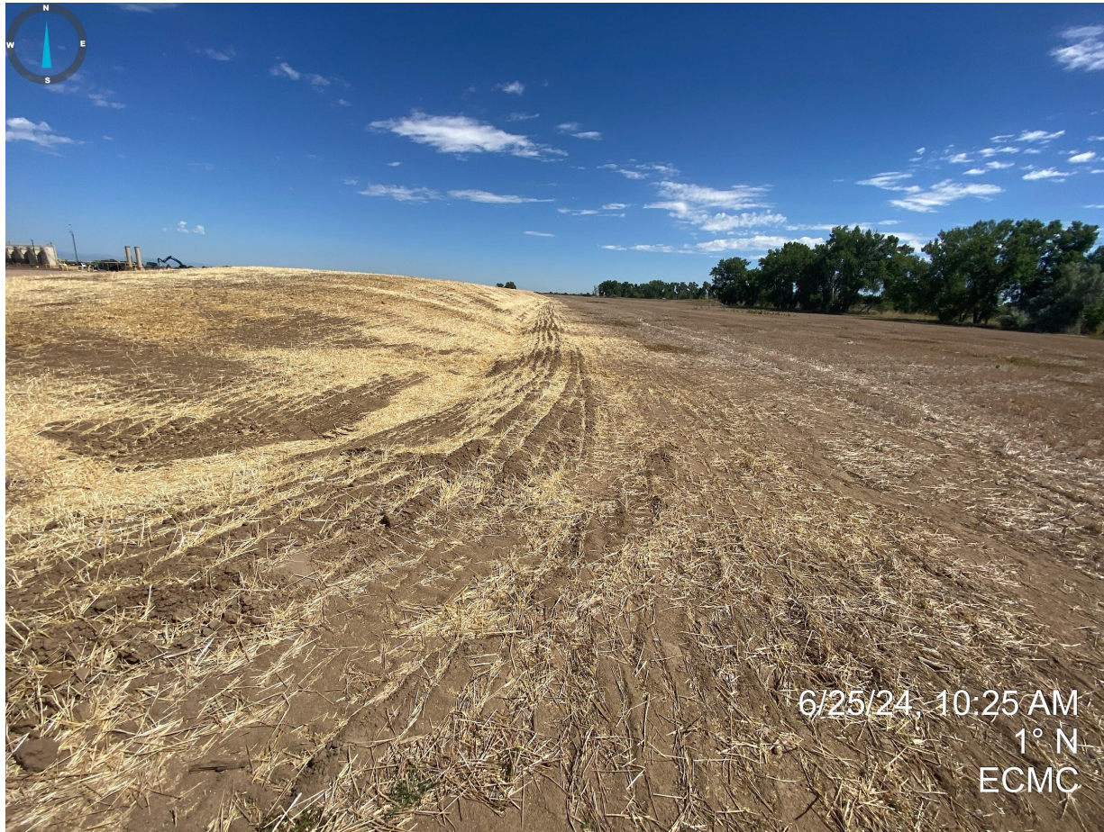
Photo 4. Southeast corner of the location. Perimeter stormwater ditch and berm, and topsoil stockpile pictured.
