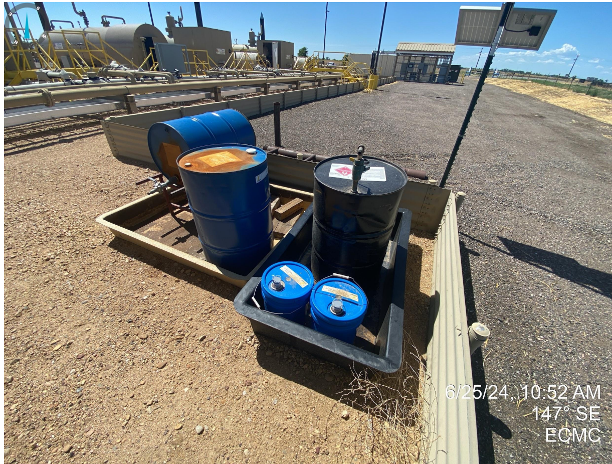
Photo 27. No wildlife netting observed around secondary containment on west end of location.
