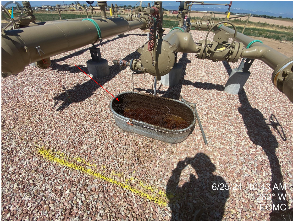
Photo 15. Netting does not appear to have been repaired since the previous inspection. Additionally, free fluids observed within secondary containment need to be properly disposed of.
