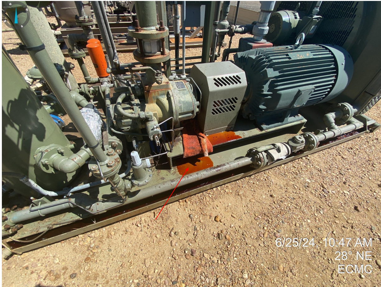
Photo 22. Free fluids observed within compressor skid on west side of location.
