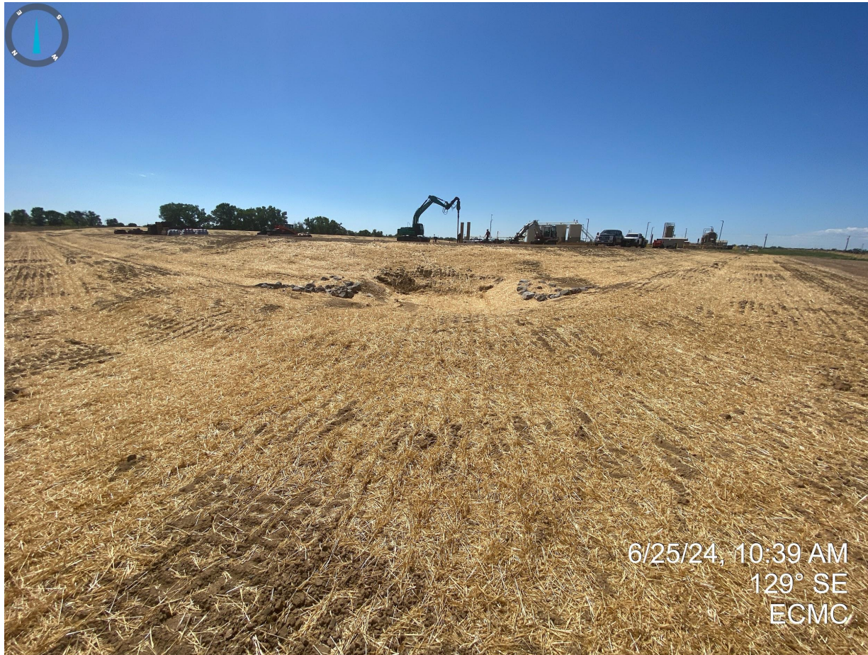
Photo 12. Sediment trap and ditch and berm installed on the northwestern portion of the construction area.
