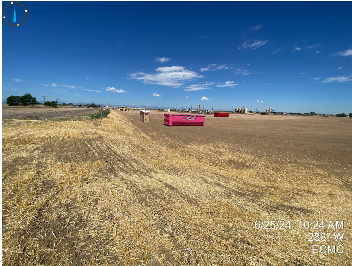
Photo 2. Southeast corner of the drilling pad. Stormwater BMPs appear to have been repaired and slopes have been stabilized with crimped mulch observed.
