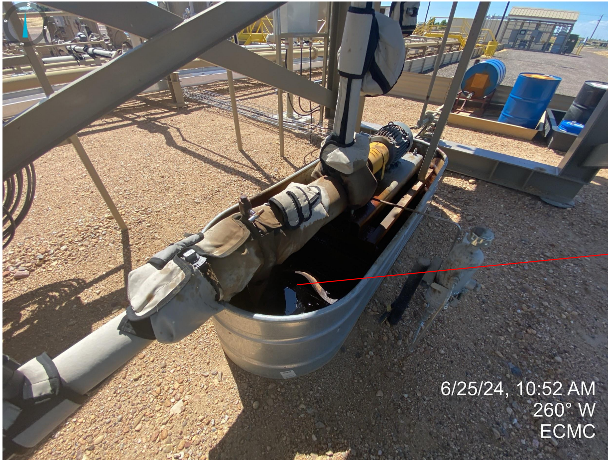
Photo 28. No wildlife netting observed around secondary containment on west end of location. Additionally, free fluids need to be properly removed and disposed of.
