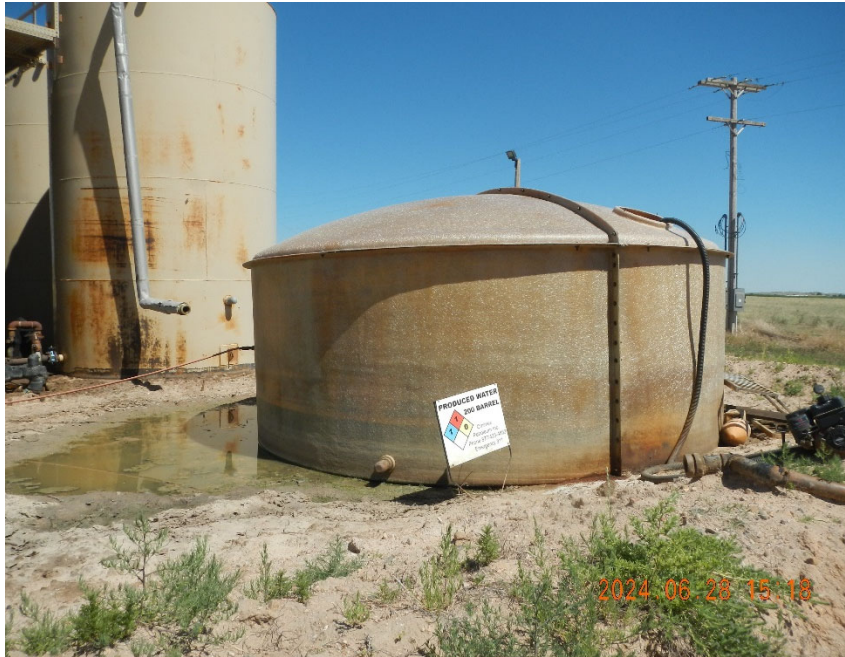
9. View of 200 BBL Fiberglass AST. Note vegetation, fluids, and equipment.
