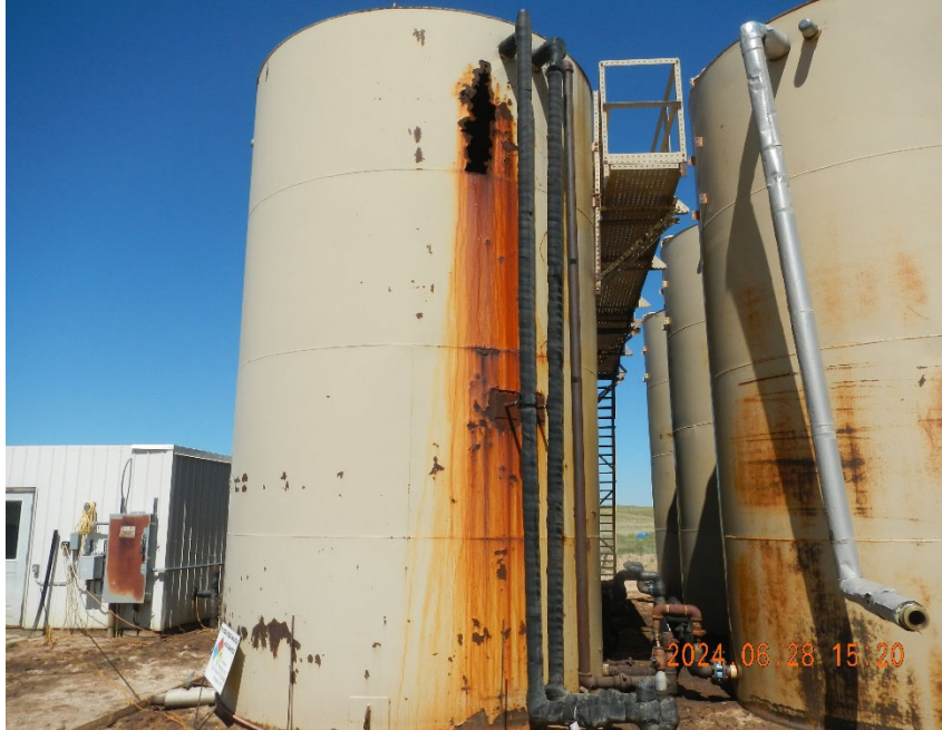
11. Steel AST has hole rusted through wall of tank.
