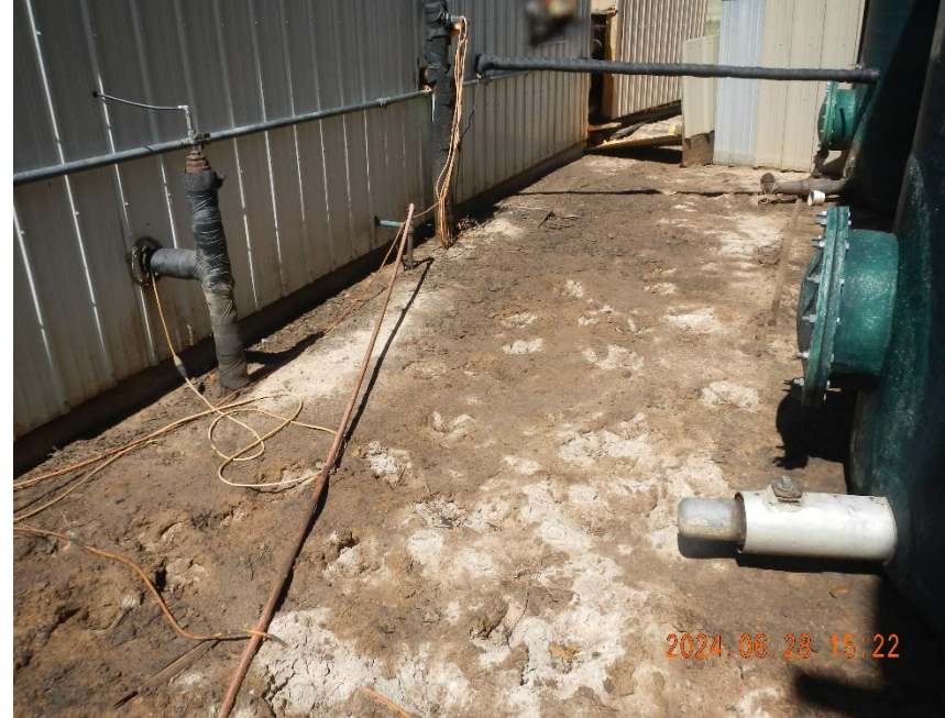
14. Additional view of soil staining inside berms. Staining is present throughout the inside of the bermed containment area.
