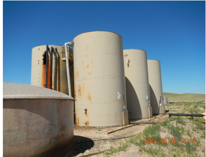
10. View of 400 BBL Steel AST's. Note vegetation and visible rust on tanks.
