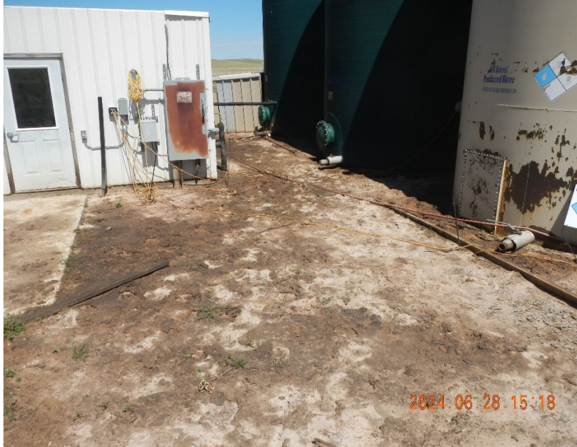
13. Visible staining of soil and concrete inside berms at tank battery.
