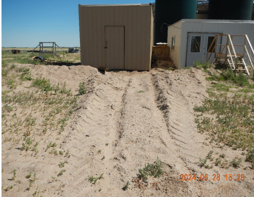
17. Containment berm opened up in front of Injection Pump making the berm inoperable as a BMP.
