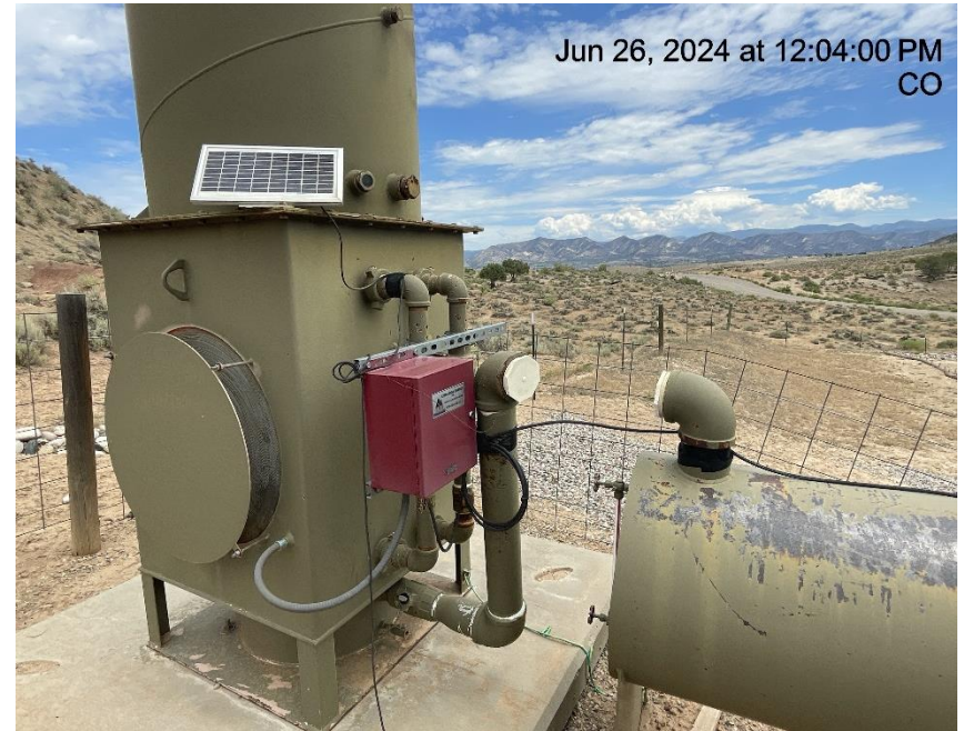
Photo # 1603 Unused equipment – ECD disconnected & not in use
