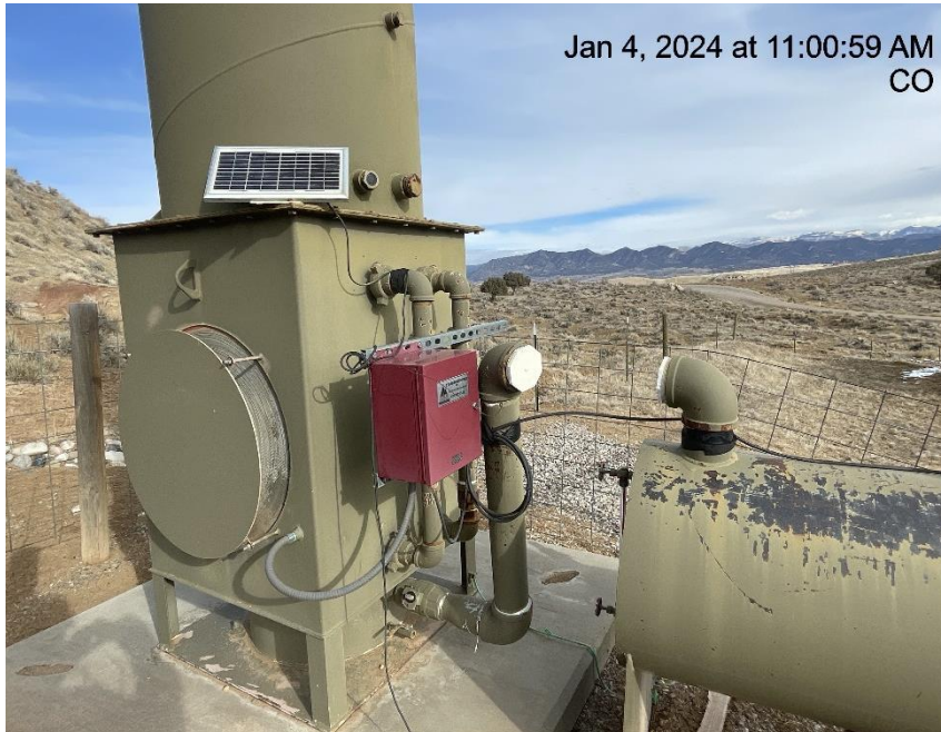
Photo # 1727 From inspection 708902717 conducted on 01/04/2024 Unused equipment – ECD disconnected
