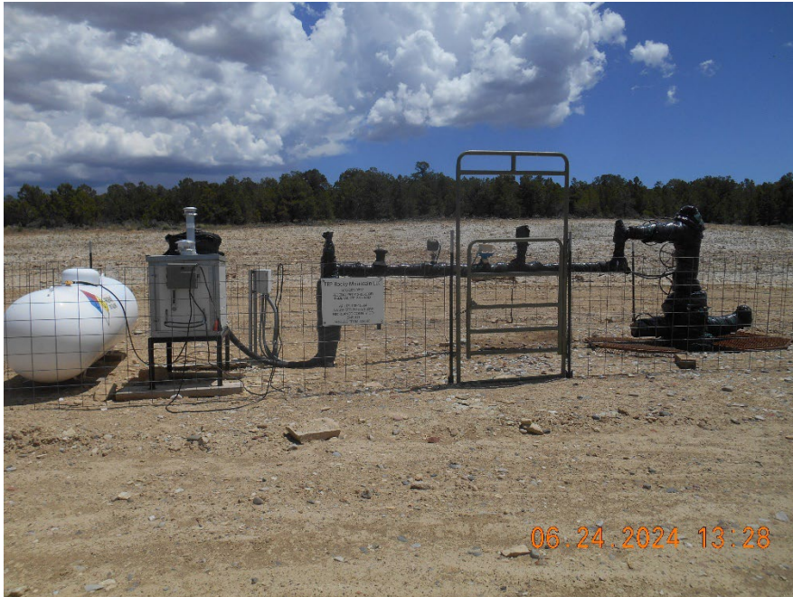
Injection wellhead and line heater
