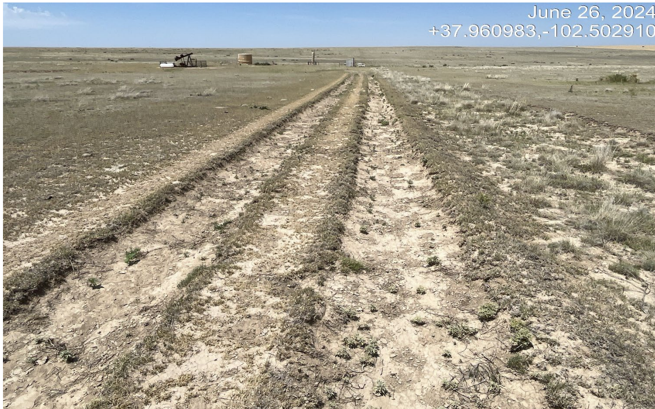
Photo 1. Facing east along the access road. There are deep ruts in the road and there are now vehicle tracks driving off the two track which is widening the road. The vehicle ruts need to be repaired and stabilized.
