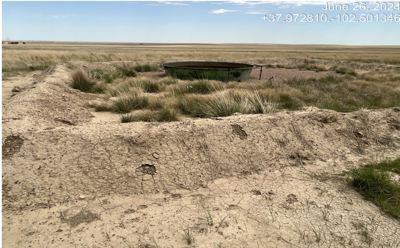
Photo 2. Facing toward the open top tank where deceased birds were previously observed. The berm has been built up better for secondary containment and netting has been placed over the tank.
