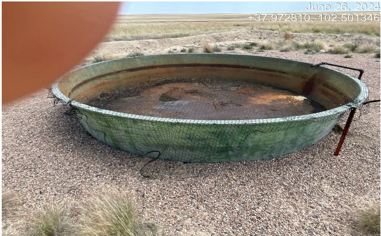
Photo 3. Netting nor covers the tank to prevent wildlife entry. There is still no labels on the tank..
