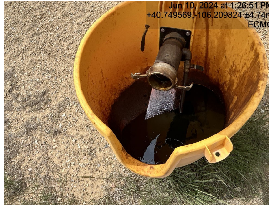
Load line missing cap/plug
